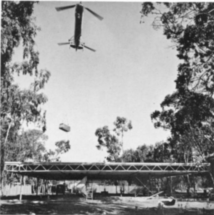
SCSD school under construction.
