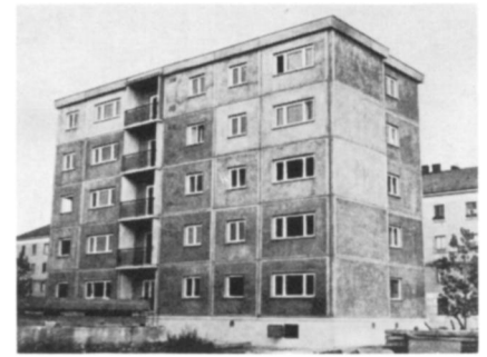
Precast panel building in Hungary.
