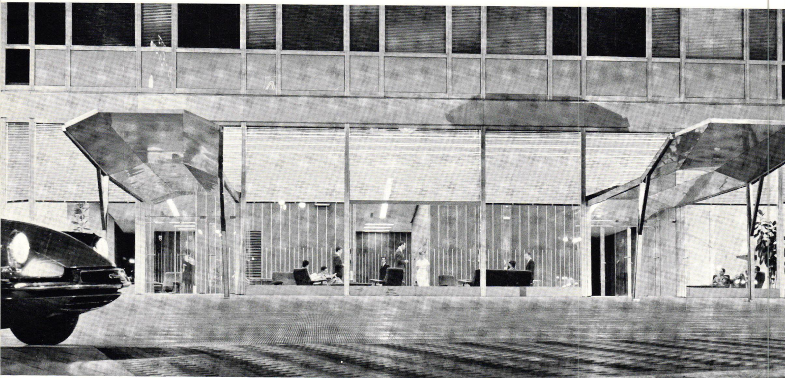
96. Main entrance canopies
