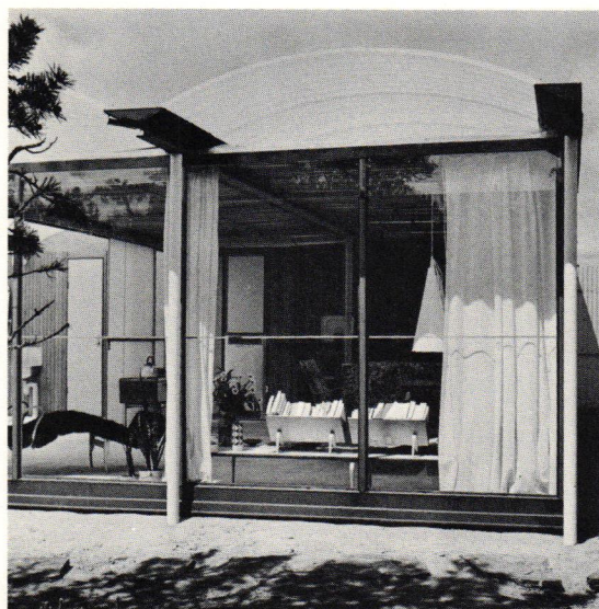
terior view showing arched roof of acrylic plastic. Interior ceiling of diagonal wood lathing (right)
