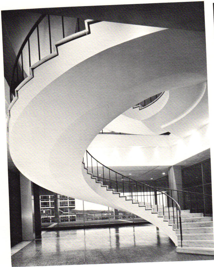
U.S. Airforce Academy Library Staircase, Colorado Springs, Colo., designed by Skidmore, Owings & Merrill, 1963
