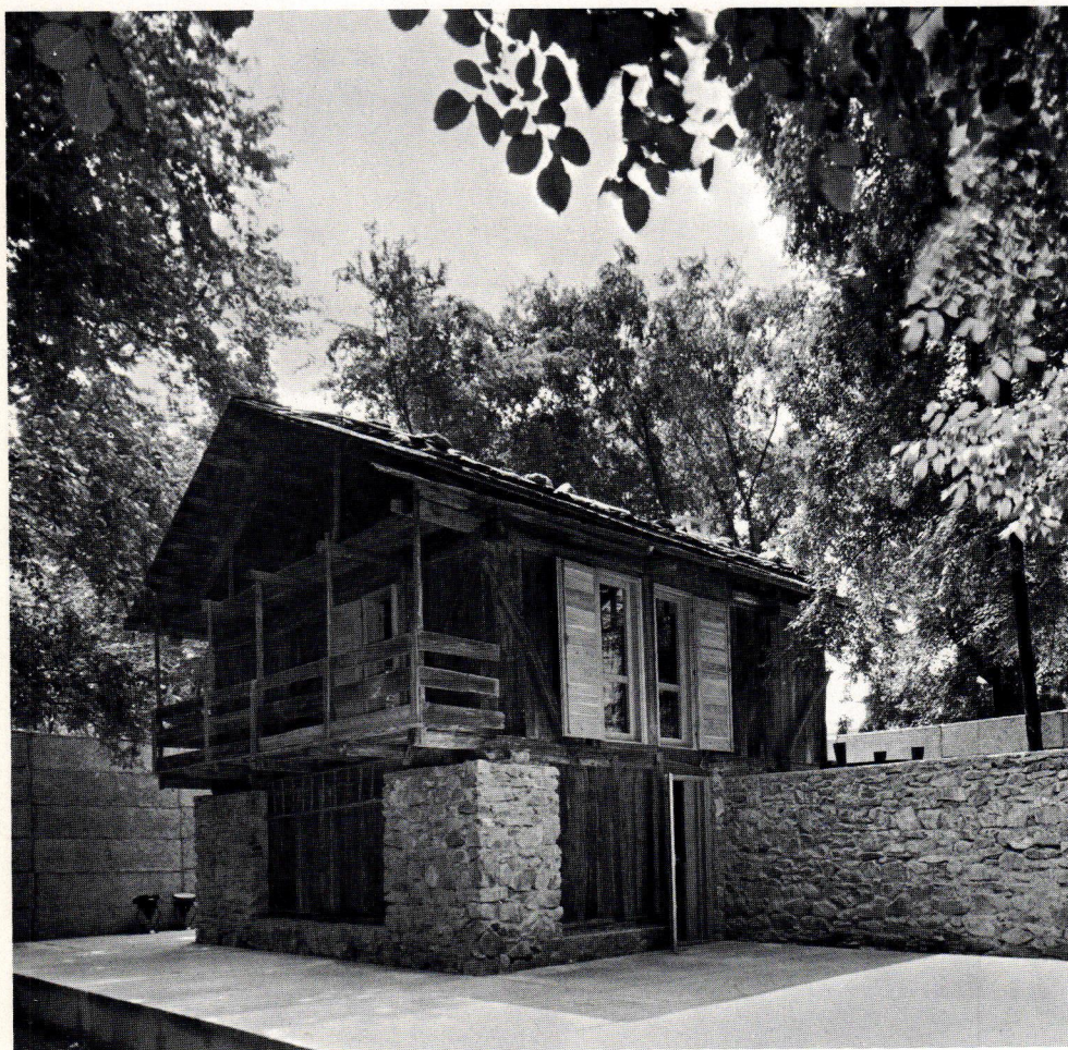
Alpine Cottage from the Trento region restored by architect S. Giovanazzi and Studio Albin and Helg.
