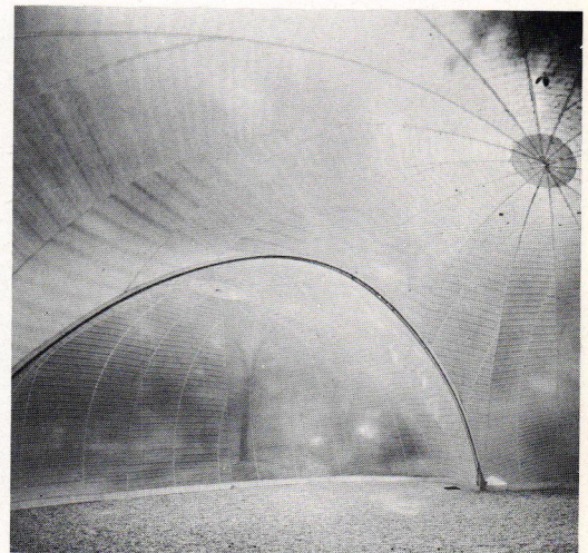
Translucent plastic dome, inflated and kept at a constant air pressure by an electric ventilator. Made by Plasteco, Milano.
