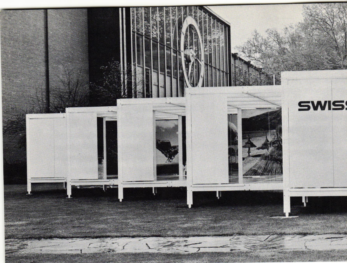
82. 83. 84. Swissair information stand. Can be assembled in various sizes and shapes; floor and ceiling panels are of equal size. The basic unit measures 10' x 10' x 10'. Steel supports are bolted into place and stairs are bolted to the coupling element between floor panels. Easily transported, the stand can be assembled by five men in one day. D: Andreas Christen, Zürich, 1959-1960
