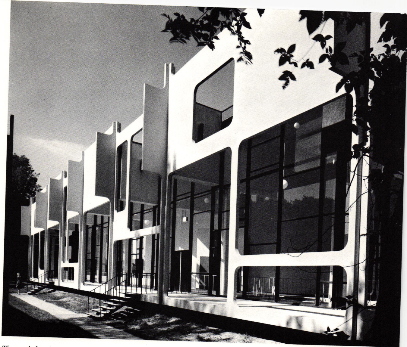
The south facade, because of the sloping site, is only one story high, whereas the north or main facade is two full stories high.
