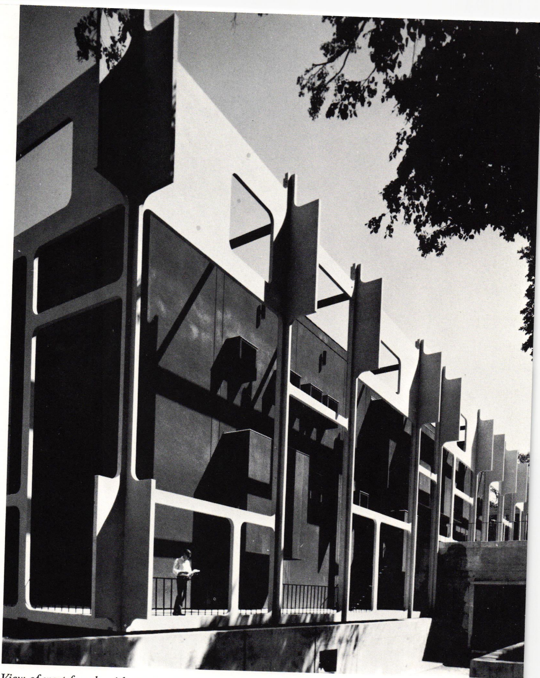
View of west facade with stage entrance and delivery door.
