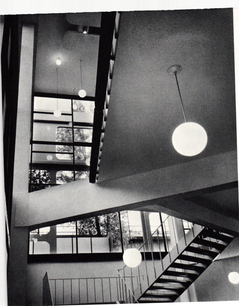
Stairs leading from entry level to balcony level. Note typical connection between balcony floor beam and column, and exposed "fin-tube" radiators on face of balcony.
