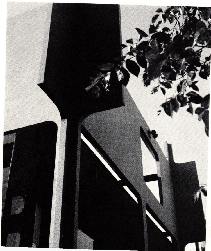
Southeast corner detail showing intersection of exterior screen.
