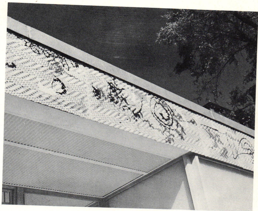
gyorgy kepes: Enamel and steel fascia for the facade of the Fitchburg Youth Library, Fitchburg, Mass. In cooperation with Karl Koch, architect.
