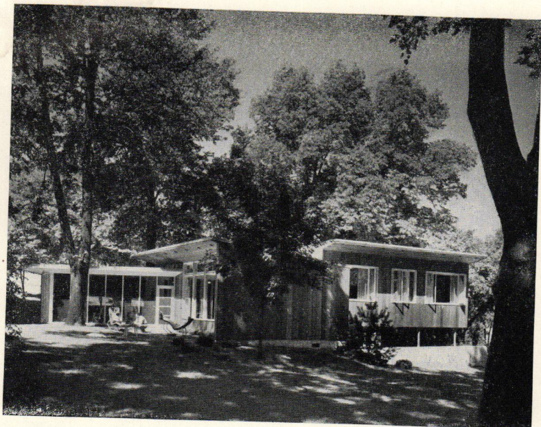
(above) Looking at the Idea House from the southeast, screened porch, terrace, and living room windows are at the left; bedroom wing at right, with carport below. The ten-inch wide vertical redwood siding has been treated with an oil preservative which protects its natural deep red color. All trim is white; gutters, roof edge and pipe columns are painted aluminum.
