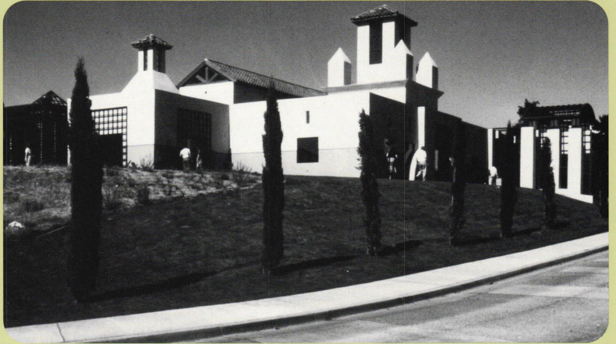
Spanishland persists as a theme in southern California architecture today. San Juan Capistrano Public Library, designed by Michael Graves, 1983.
