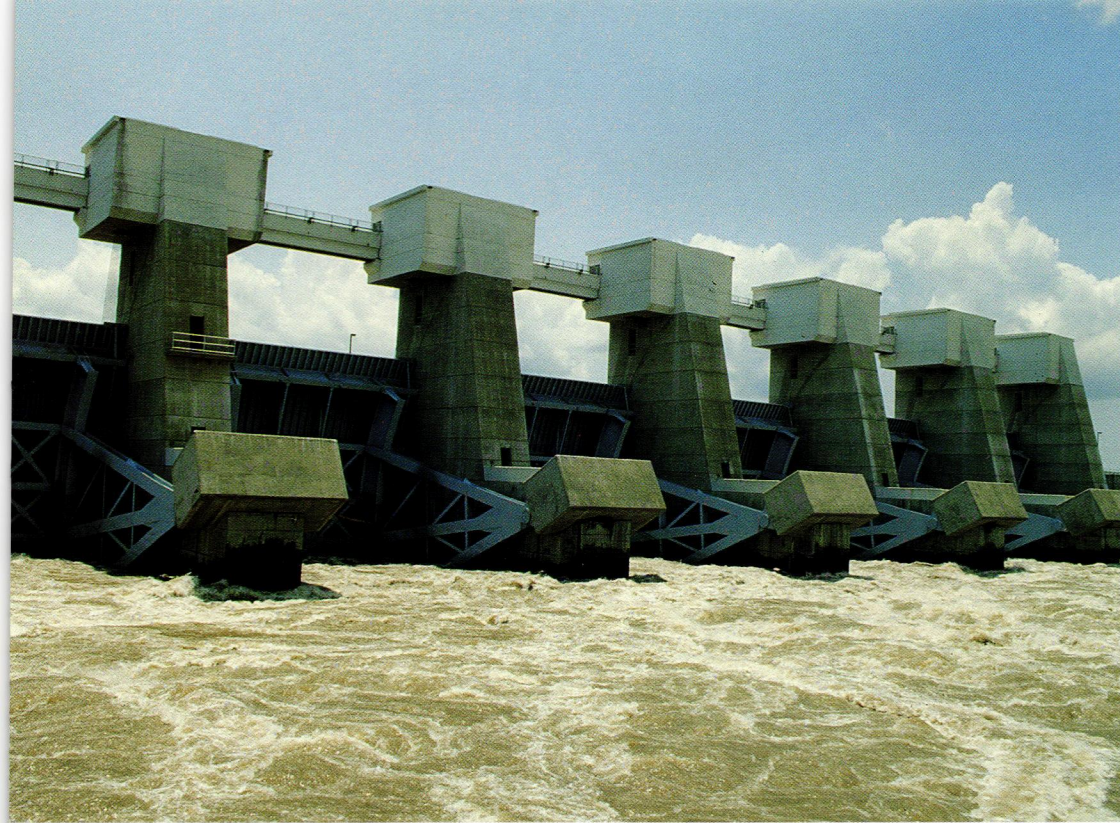
Old River Control Structure, Louisiana
