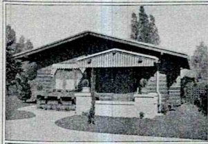
The Cement Porch Adds an Artistic Touch to This Bungalow
