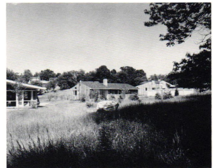
(from top) Case Study House #8 by Charles Eames, 1949, is located with three other Case Study Houses on Chautauqua Way in Pacific Palisades, California.
