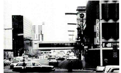
17 3rd Avenue looking north at the connection between Norwest Service Center and the Gateway Municipal Ramp, Minneapolis, 1985
