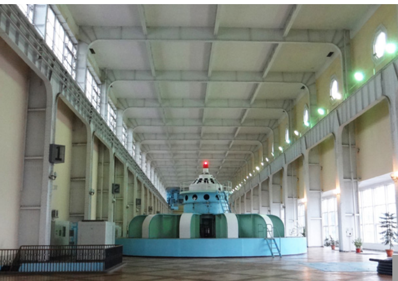
05 Interior of the hydroelectric station. © S. Smolenska, 2017.
