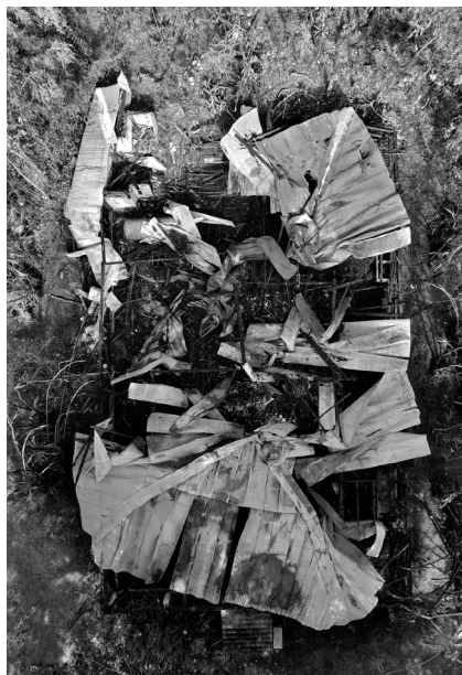
01 Casa Klumb, aerial fire detail. © Javier Olmeda, 2020..
