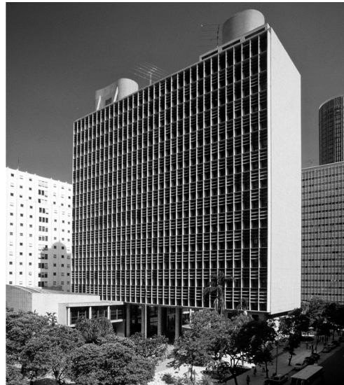
sections: operable brise-soleil
