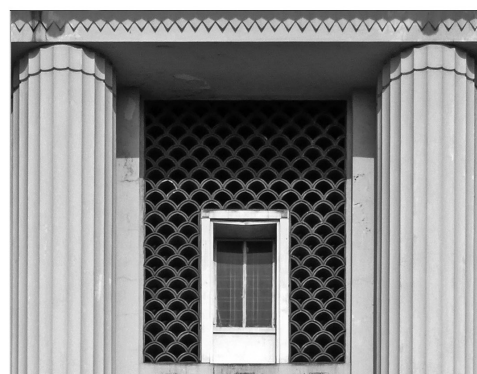
01 Rangoon Jalis . Top right: T. O. Foster, Port Trust Offices, Rangoon, Burma, 1926-1930 – described in Basil Ward's Rotary Club speech. First use in 1930 of innovative glazed terracotta sun-screening. Left and bottom right: Basil Ward for T. O. Foster, National Bank of India, Rangoon, Burma, 1929-1932, probably designed and completed by Basil Ward. Photographs © Pedro Guedes.
