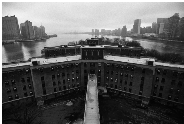
03 Isadore Rosenfield with Kohn & Butler, Yorke and Sawyer Archs, Goldwater Hospital, New York, USA, 1939, view south to ward buildings A and B from administration building E. © Charles Giraudet, 2014.
