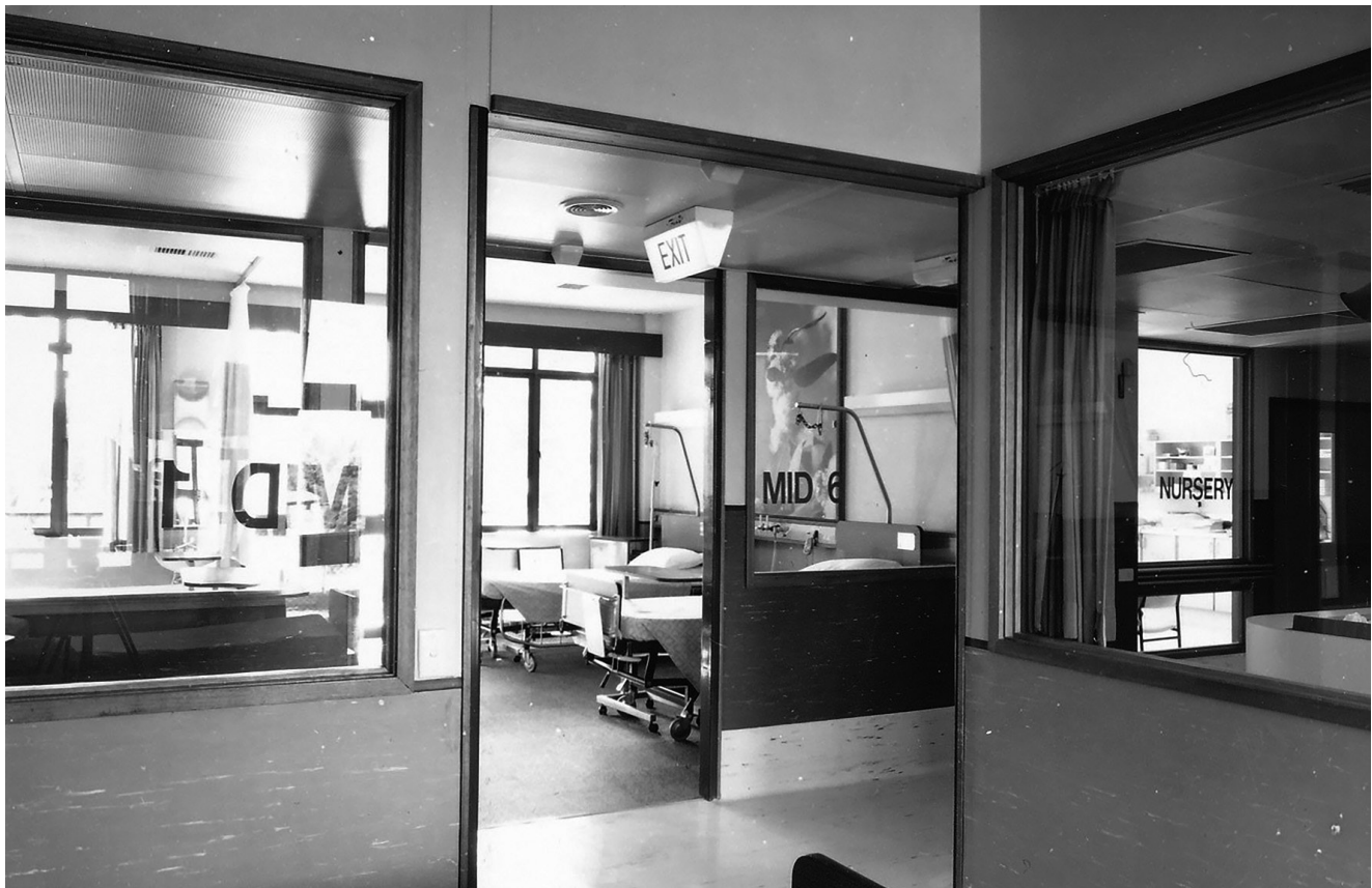
09 Interior view of Charleville Hospital (1939), typical internal arrangement whereby extensive glazing allows the penetration of natural light and ventilation. © Source: Fulton Trotter Architects Archives.
