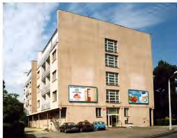
Fig. 2, Adolf Rading's Turmhaus, Breslau (now Wrocław), Germany (now Poland), 2010, view from the road, south west side, photo. W.Borski.
