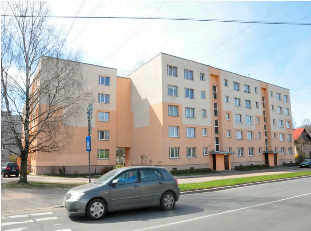
Figure 4. Housing renovation on Bebru Street, Riga, Latvia, 2017 © S. Treija
