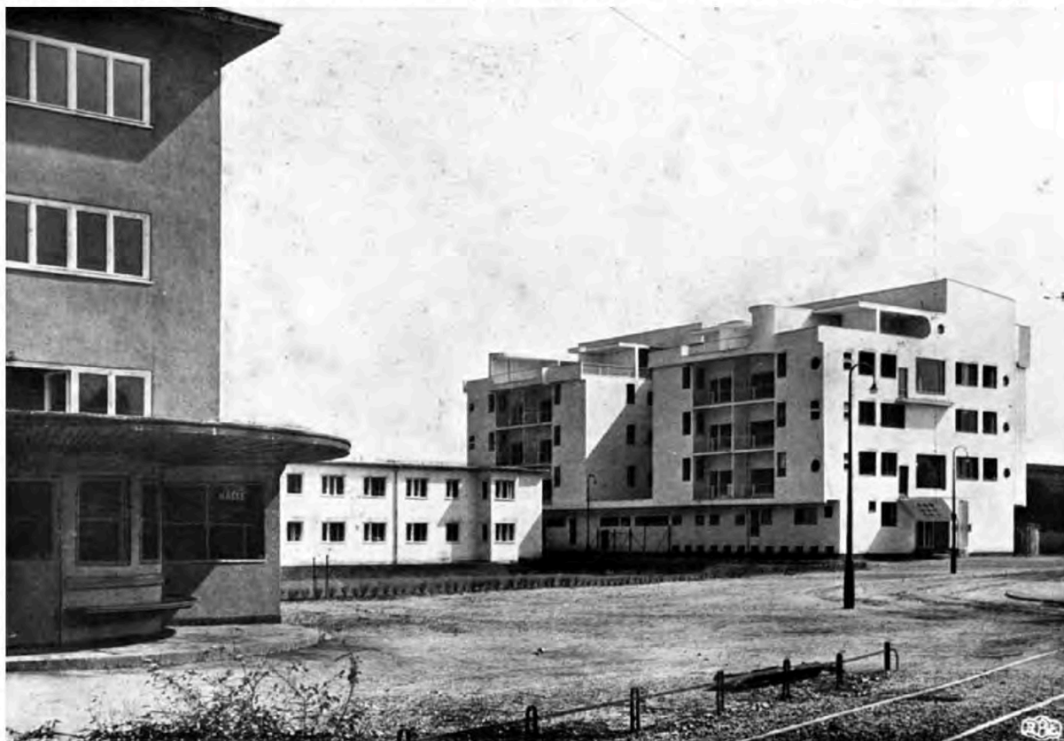
Fig. 1, Adolf Rading's Turmhaus, Breslau (now Wrocław), Germany (now Poland), 1929, view from south west, Architektura i Budownictwo , 1929, p.324.
