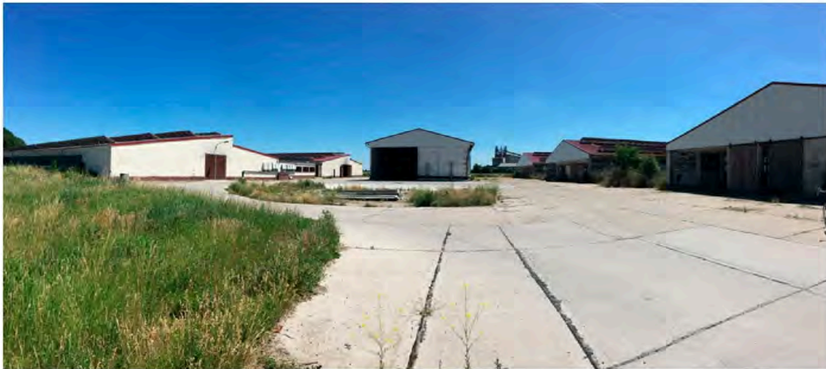
Figure 5: Stables, Golzow (South Oderbruch). © MODSCAPES, 2017.
