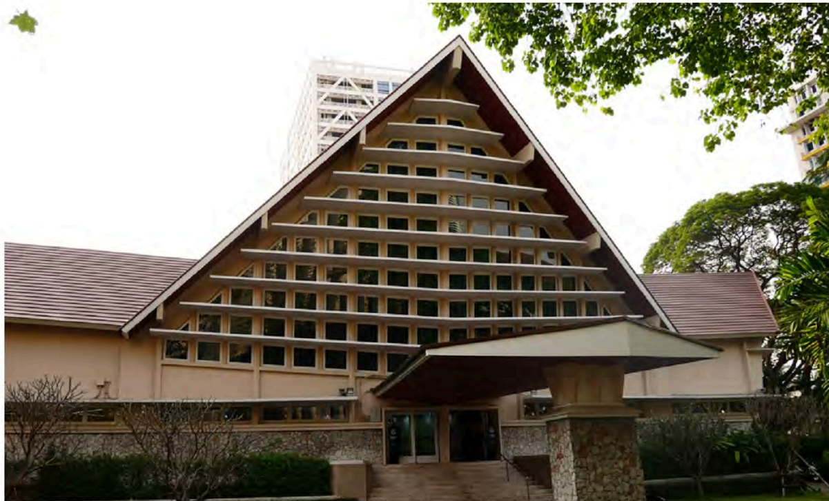
Sala Phra Kiew Building, Chulalongkorn University, Bangkok, Thailand. Photo by: Noppawan Ratanamart
