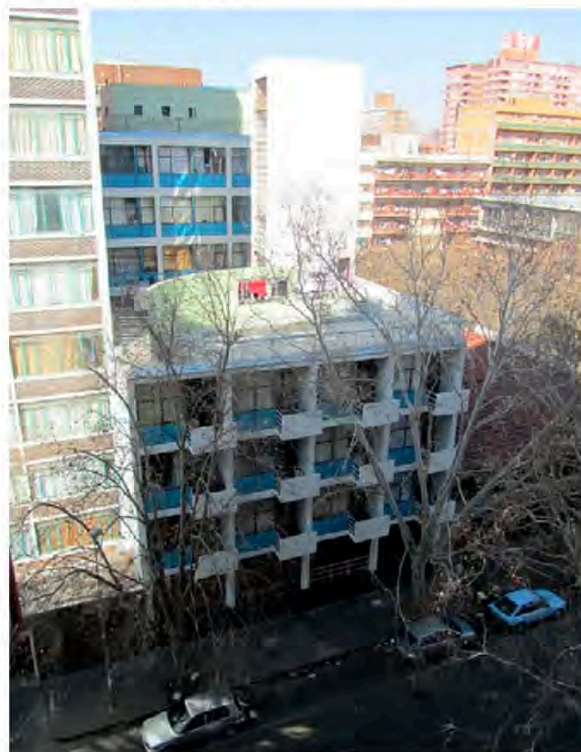
Image 4 - Detail of the modulated street facing façade with cantilevered balconies (Photograph courtesy of Mayat Hart Architects)
