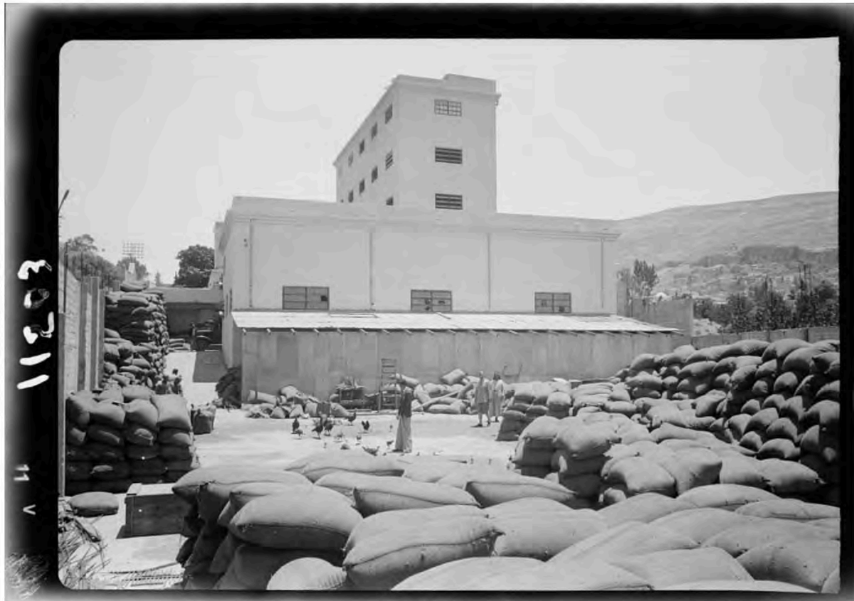
A general view of al-Na'ama Flour Mill from the west, 1940, G. Eric and Edith Matson Photograph Collection, Library of Congress, Washington DC.
