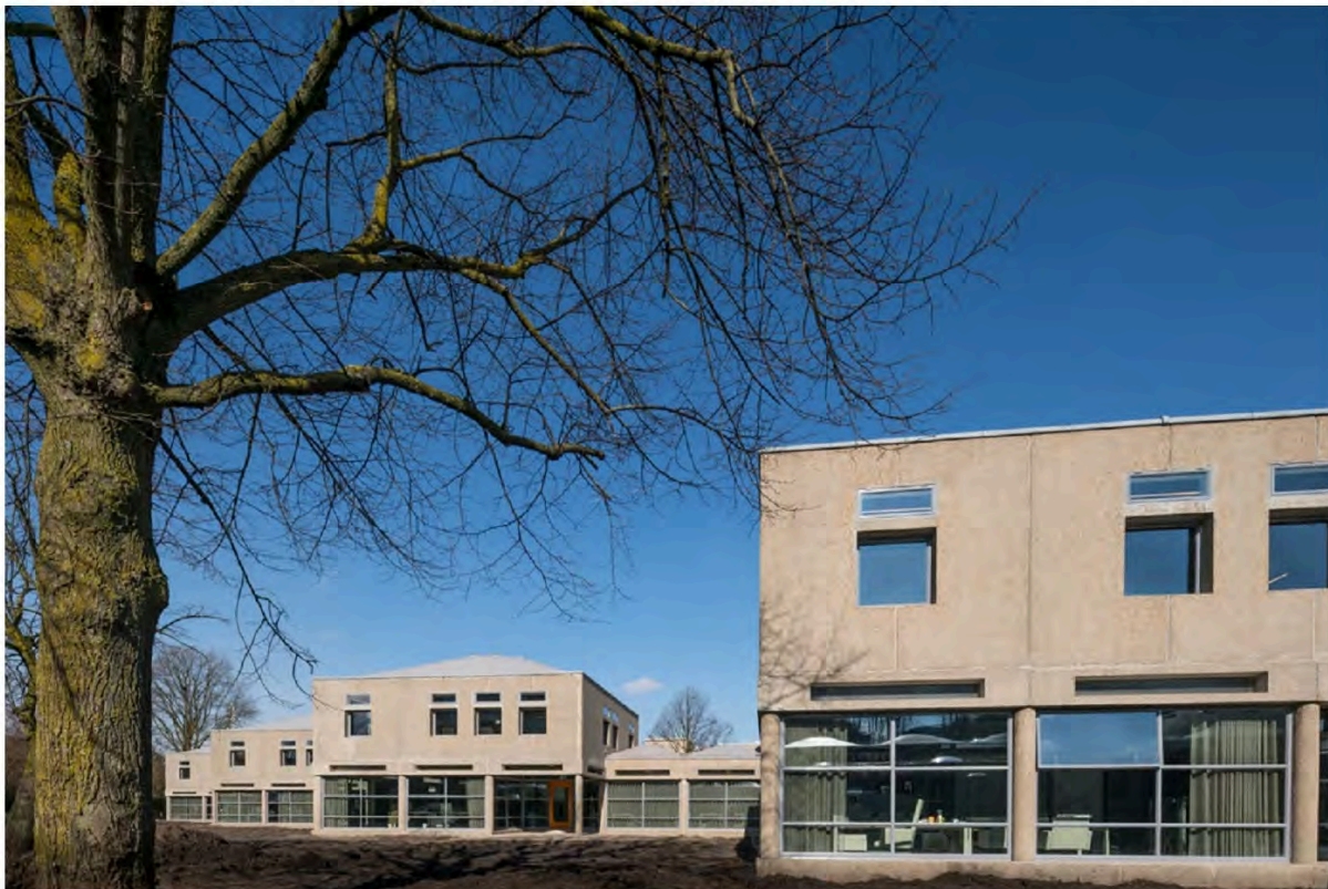
Fig. 1. Aldo van Eyck, Orphanage, Amsterdam, 1960. Overview of the four pavilions for the older children after restoration. Photo © Jannes Linders.
