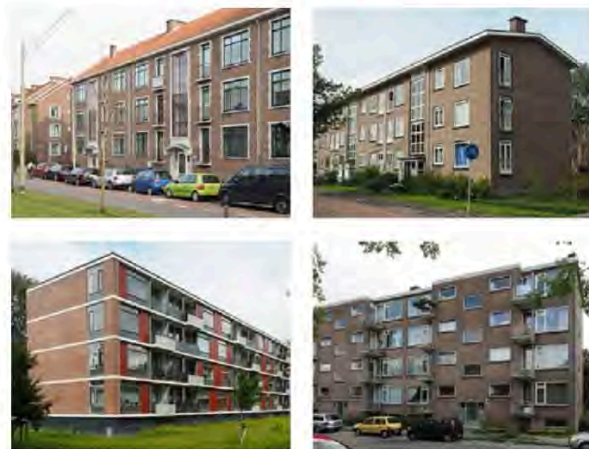
Fig. 1 Four subtypes. Top left: subtype 1 interwar traditional construction methods Amsterdam. Top right: subtype 2 interwar traditional construction methods Den Haag. Bottom left: subtype 3 postwar mixed construction methods. Bottom right: subtype 4 postwar construction systems. Pictures are from the municipal picture data banks of Den Haag Amsterdam and Utrecht.
