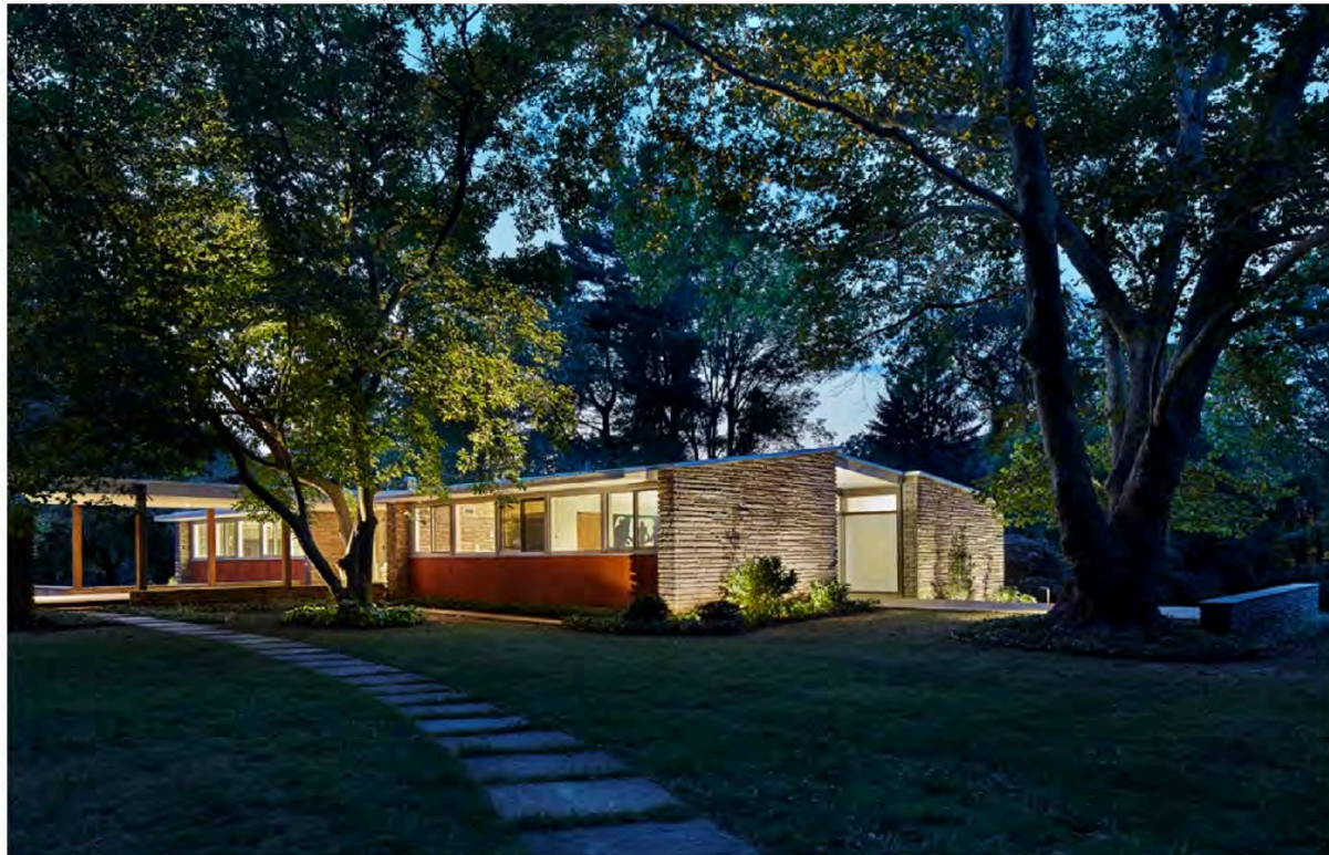
Figure 1. Vincent G. Kling, Smith Residence, Gladwyne, Pennsylvania, U.S.A, 1959, front exterior view. © Jeffrey Totaro.
