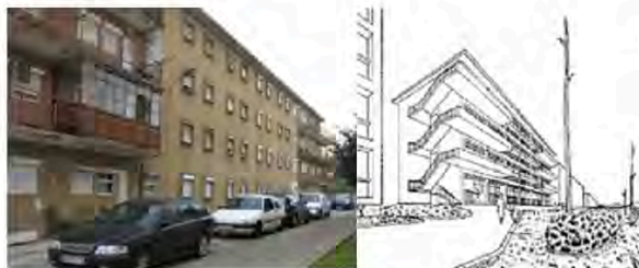
Fig. 2 CTT Housing Blocks neighbourhood, Porto, 1955. Luís Almeida d'Eça and Porto City Council.
