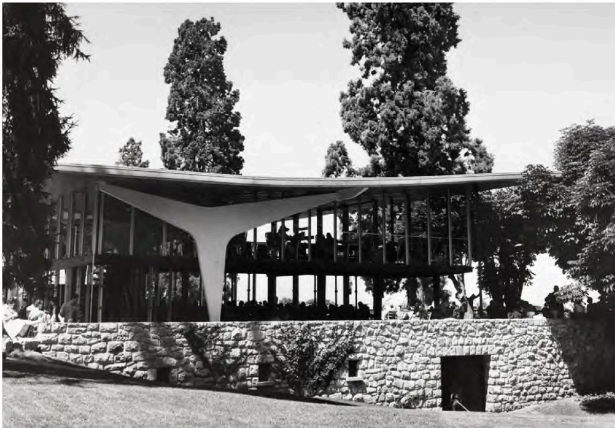
Figure 3. The Évian buvette east façade, demolished in the 1980's © ADHS.
