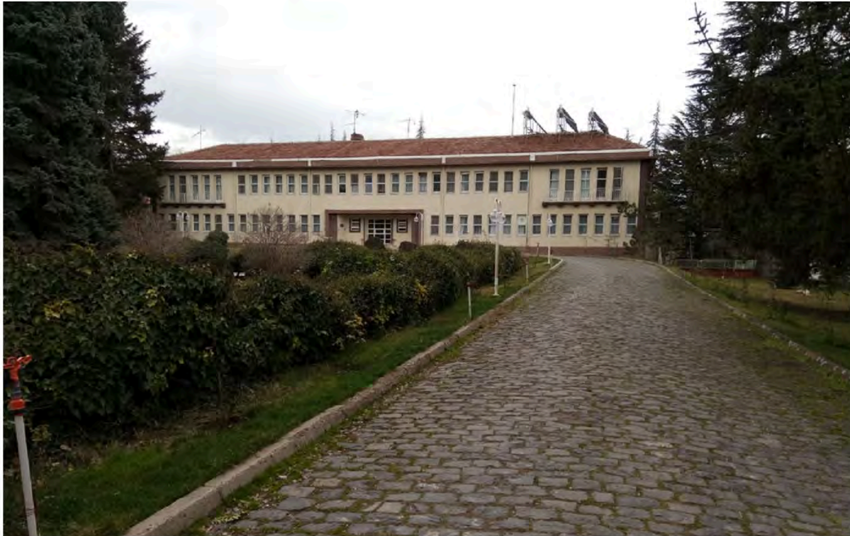
Administration Building of the Eskişehir Sugar Factory (1933). Photo by Figen Kivilcim Corakbas, 2018.
