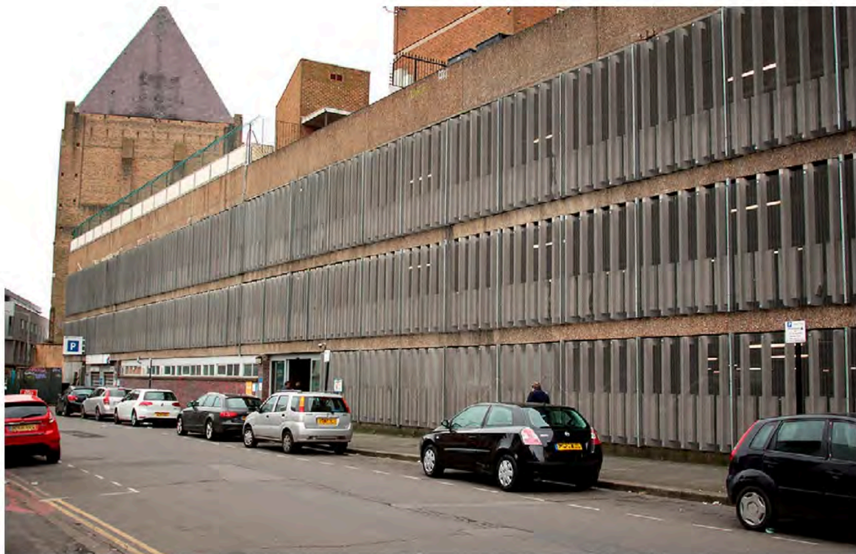
Figure 4. London Road Car Park, Brighton & Hove, United Kingdom, Façade. https://electricbrighton.com/london-road-car-park
