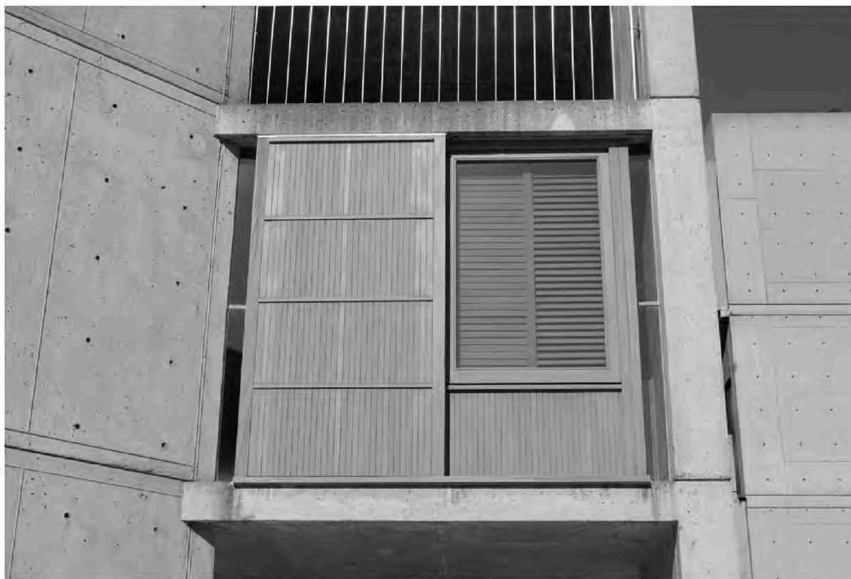
Figure 3. Salk Institute for Biological Studies, La Jolla, California, USA, 2017. View of conserved window wall assembly in the north study towers. © Wiss, Janney, Elstner Associates Inc., 2017.
