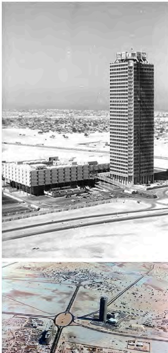
Fig. 2. John R. Harris and Partners, National Bank of Dubai, Dubai, UAE, 1979. © John R. Harris and Partners
