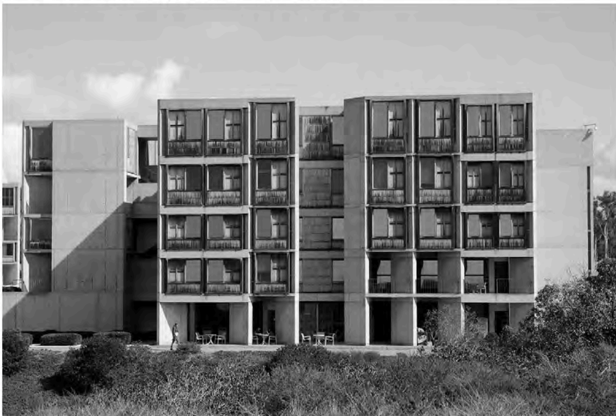
Figure 2. Louis I. Kahn, Salk Institute for Biological Studies, La Jolla, California, USA, 1965. View of west-facing office wing, illustrating black fungal biofilm at base of window wall assemblies prior to conservation. © J. Paul Getty Trust, 2013.
