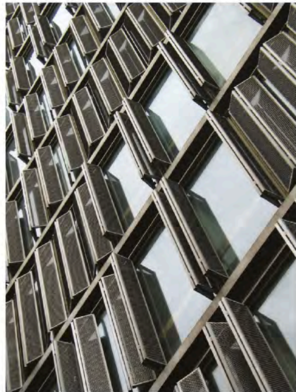
Figure 3: Left: Axonometric view of a window panel showing all the pieces that were dismantled for cleaning or replacement. © P. Roux, 2015. Right: Aluminium shutters and post-and-beam apparent steel structure. © K. Kramski, 2014.
