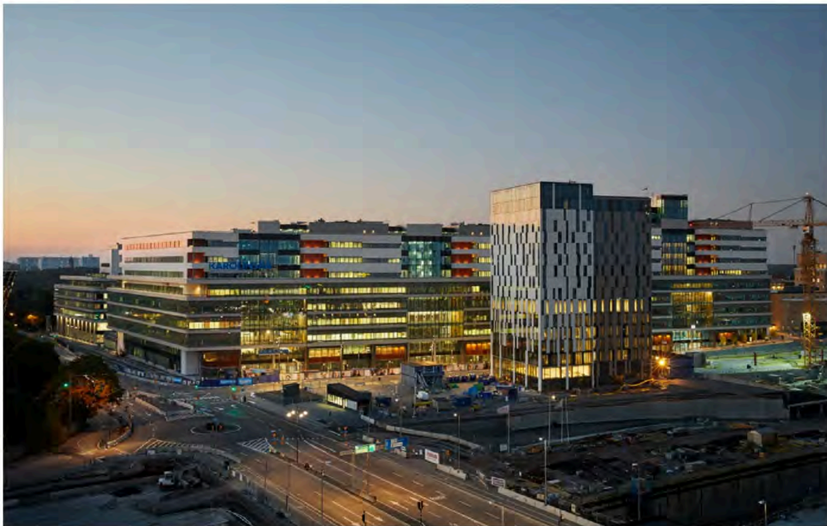
New Karolinska Hospital in Solna 2018. White architects’ largest project ever with a high degree of flexibility.
