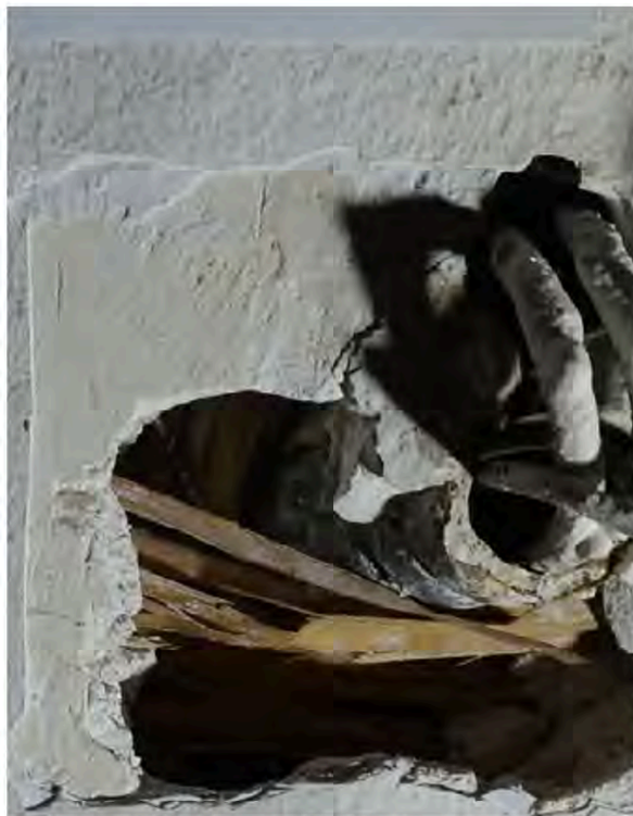
Figure 3. Villa Beer, 1930, Vienna, Austria: music gallery, ceiling, the original yellowish-white paint uncovered. © Ivo Hammer, 2017
