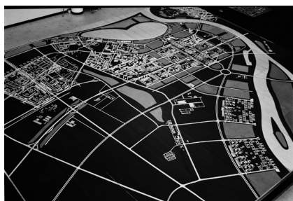
03 Urban Planning Institute of Belgrade, New Belgrade, Belgrade, SFR Yugoslavia. Modular working-model per plan of 1962 on display in the Institute for Construction of (New) Belgrade – scale models would be inserted after the adoption of the detailed urban plan for each urban block. Most of the depicted blocks were built as designed per these plans. © Urban Planning Institute of Belgrade, c. 1970.
