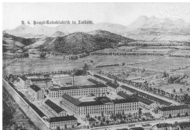
03 Tobačna Tovarna [Tobacco Factory], Ljubljana, 1873. Typical industrial architecture of the 2 nd half of the 19 th century, situated on the city outskirts, next to the railway. Built in a brick external structure, with an internal system of cast iron columns and beams. © Sonja Ilko.
