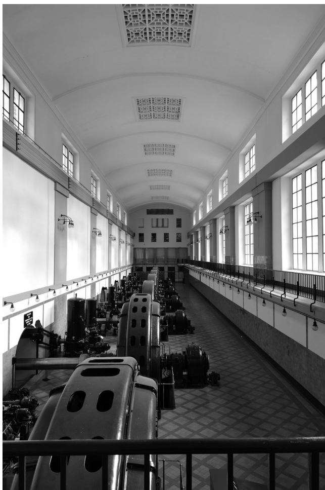
04 E. Faesch, Power House, Fala hydropower plant, 1918, with an innovative inside shell ceiling, only 5 cm thick, has been renovated into a museum, partly still operating with new generators. This is a case of symbiosis between heritage protection and the industry. © Miran Kambič.
