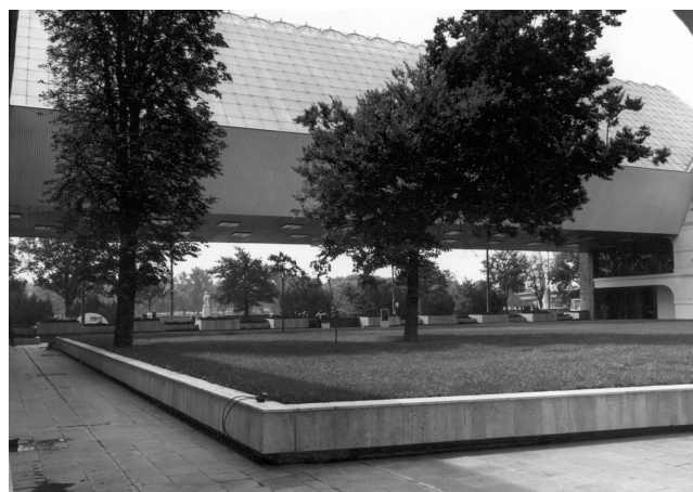
06 Vladimír Deděček, Slovak National Gallery, Bratislava, Slovakia, 1967-1979. View from the courtyard to the glass roof of the exhibition block. © Archive of Department of Architecture HÚ SAV.
