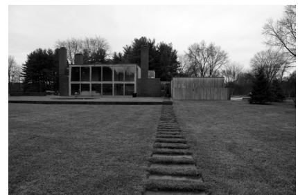
01 Louis Kahn, Korman House, Whittemarsh Township, Pennsylvania, USA, 1971–1973. © Ana Tostões, 2018.
