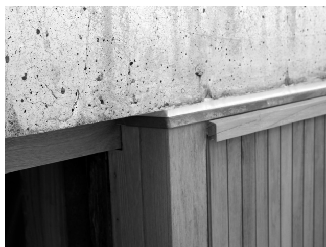
09 Louis Kahn, Salk Institute, La Jolla, California, USA, 1959-1965. Folded metal flashing installation at top of window. © Wiss, Janney, Elstner Associates, Inc. 2016.
