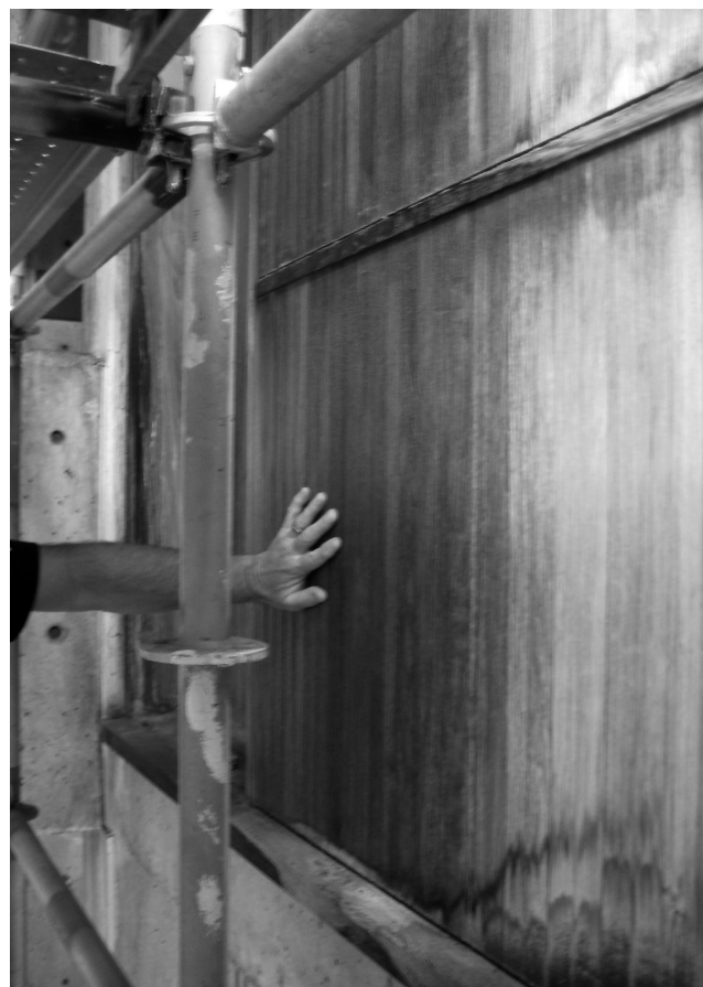
07 Louis Kahn, Salk Institute, La Jolla, California, USA, 1959-1965. Treatment discoloration and varied weathering patterns. © Wiss, Janney, Elstner Associates, Inc. 2015.
