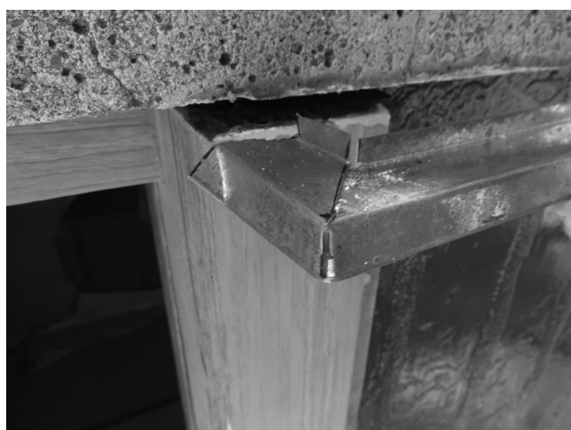
08 Louis Kahn, Salk Institute, La Jolla, California, USA, 1959-1965. New metal flashing at top of window. © Wiss, Janney, Elstner Associates, Inc. 2016.
