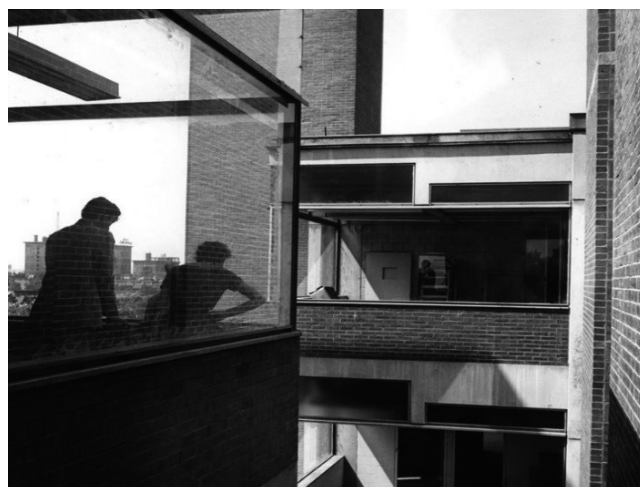
04 Louis Kahn, Richards Laboratories, Philadelphia, USA, 1957–1961. View between two towers showing stainless steel glazing frames. © Mildred Schmertz Photograph, University of Pennsylvania Architectural Archives, 1961.
