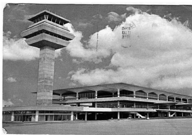
05 Kingston Loo of BEP, Kuala Lumpur International Airport, Subang, Malaysia, 1965. With a hyperbolic paraboloid concrete roof and the longest runway in Southeast Asia at the time of its construction, the airport was as one of the most modern airports in the region in the 1960s. © National Archive, 1960s.
