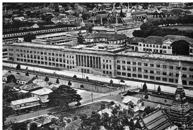
04 Saroj Sukhyanga, Ministry of Justice, Bangkok, Thailand, 1940. This important building was demolished in 2013. © Chatri Prakinnonhakarn, Seminar paper on Supreme Court demolition, Bangkok, Faculty of architecture Silpakorn University, 2013.
