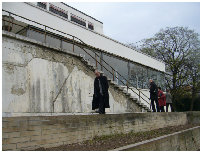
08 Mies van der Rohe and Lilly Reich, Tugendhat House, Brno, Czech Republic, 1929-30. Garden stair case, before restoration: stability problems and rests of original façade plaster and later coatings, garden walls reconstructed in 1970 using carved stones. © Ana Tostões, 2009.
