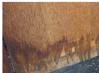
05 Mies van der Rohe, Carr Memorial Chapel, Chicago, Illinois, 1952. Damage at the bottom of wood veneer panel due to improper cleaning methods and UV degradation. © Harboe Architects, 2011.
