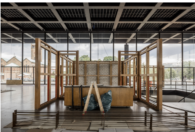
07 Mies van der Rohe, Neue Nationalgalerie , Berlin, Germany, 1968. Refurbishment by David Chipperfield Architects, 2017. The original cloakrooms in the upper hall are fully dismantled. The repair of the wooden paneling will be executed in a workshop environment. © Ute Zscharnt for David Chipperfield Architects, 2016.
