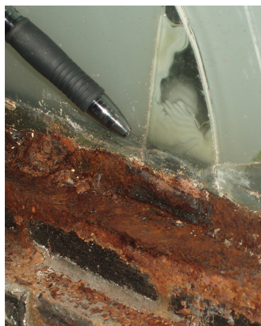
07 Mies van der Rohe, Crown Hall, Chicago, USA, 1950-1956. Detail view of sill with glazing stop removed. © Krueck + Sexton, 2005.
