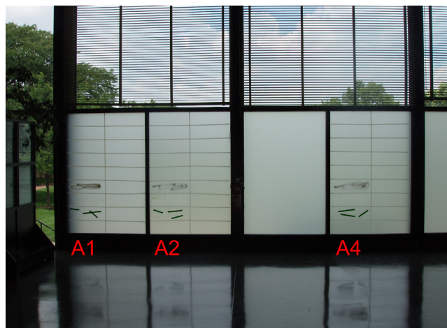
08 Mies van der Rohe, Crown Hall, Chicago, USA, 1950-1956. Mock-up sample of various materials on glass to test seal. © Krueck + Sexton, 2004.
