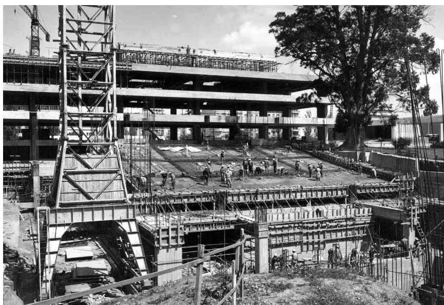
05 Alberto Pessoa, Pedro Cid, Ruy Jervis d'Athouguia, Calouste Gulbenkian Foundation, Lisbon, Portugal, 1959–1969, auditorium construction. © FCG Archive, 1966.
