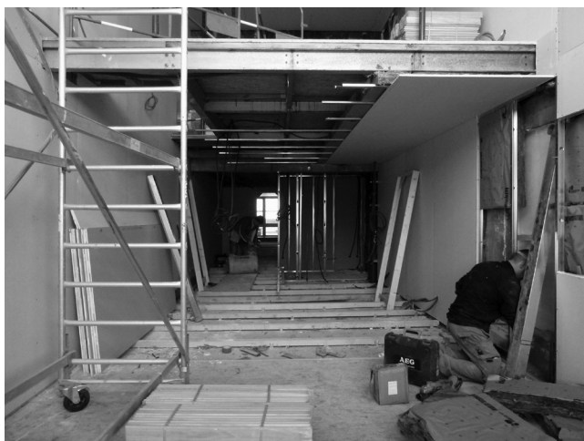
06 Le Corbusier, Unité d'Habitation , Marseille, France, 1945-1952. Reconstruction of fire-damaged apartments. Installation of the firewall partitions of precast gypsum panels. © Photo F. Botton/ssea, March 2014. FLC/2016, ProLitteris, Zurich.
