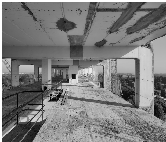
04 Willy Van Der Meeren, Ieder Zijn Huis , Brussels, Belgium, 1953–1961. A typical storey dismantled during renovation. © ORIGIN, Georges De Kinder.
