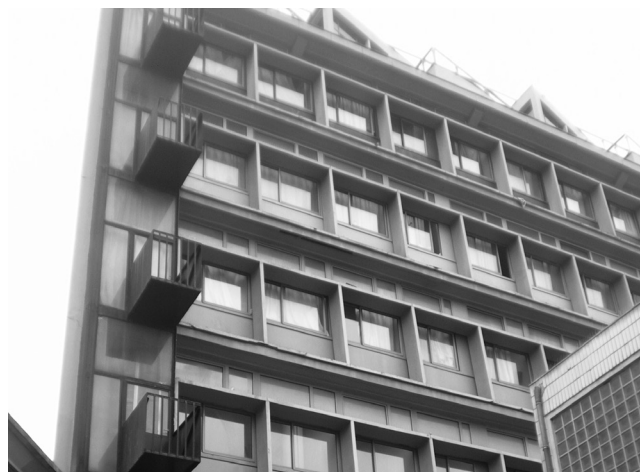
04 Le Corbusier and Pierre Jeanneret, Cité de Refuge , Paris, France, 1933. South façade before the last restoration work. On the left-hand side the slice of the original 1933 glass facade and the balconies redone at an unknown date, though after the death of Le Corbusier. © Gilles Ragot, 2012.
