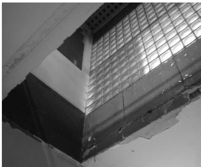
13 Le Corbusier and Pierre Jeanneret, Cité de Refuge , Paris, France, 1933. Unblocking the stair opening between the entrance hall and the ground floor below. © Gilles Ragot, 2015.
