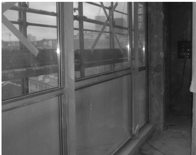
09 Le Corbusier and Pierre Jeanneret, Cité de Refuge , Paris, France, 1933. To restore the profiles of metal frames of the 7 th floor, as closely as possible to the original, a solution of invisible interior vertical stiffeners was adopted. © Gilles Ragot, January 2015.
