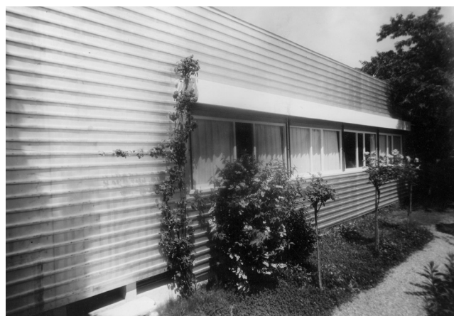
09–10 Le Corbusier and Pierre Jeanneret, Villa Le Lac , Corseaux-sous-Vevey, Switzerland, 1924. South façade before and after the metallic recovering in 1951, © FLC/SPA, 1925 (after April) and Eric Ed. Guignard, 1987
