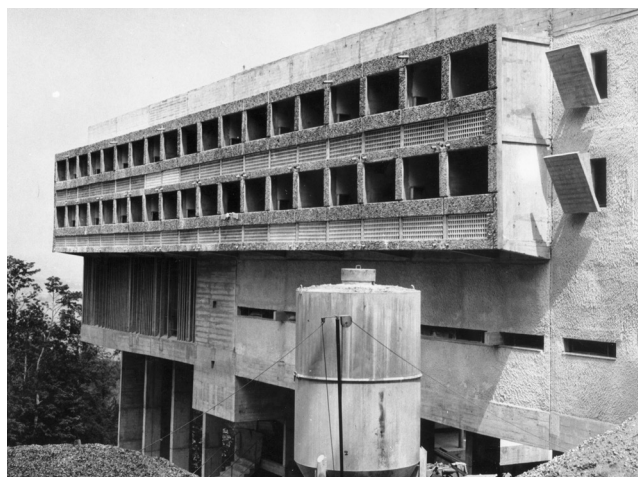
02 Le Corbusier, Couvent de La Tourette , Eveux, France, 1953–1960. The cracks on the acrotères (parapets) are already visible before the completion of the worksite. © FLC/SPA, ACT, late 1950s.
