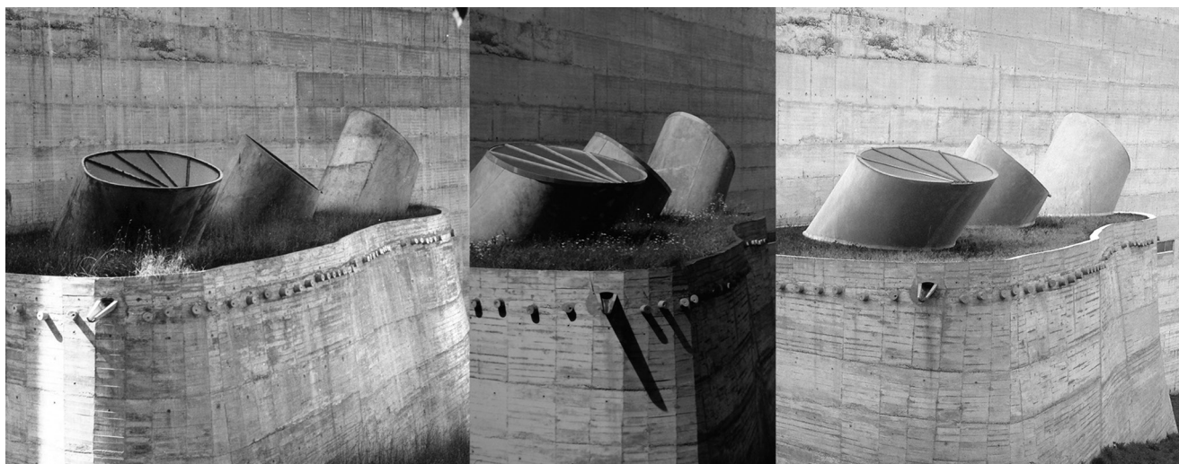
14 Le Corbusier, Couvent de La Tourette , Eveux, France, 1953–1960. The canons à lumière (skylights) of the crypt: on the left the original solution; in the center the fixtures added by the ACMH Mortamet during the first restoration, on the right the fixtures after the last intervention. © FLC/ADAGP; left: FLC, centre: Carolina Di Biase; Right: Roberto Grignolo.
