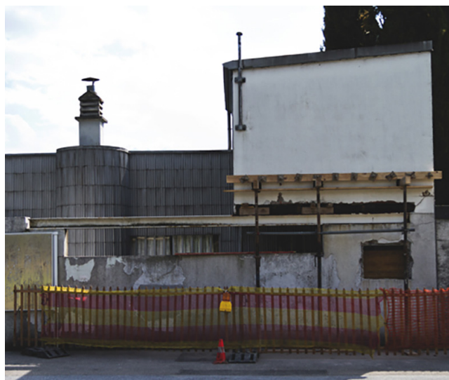
05 Le Corbusier and Pierre Jeanneret, Petite Maison , Corseaux, Switzerland, 1924. The original steel I-beam after restoration. © Giulia Marino, 2014.
