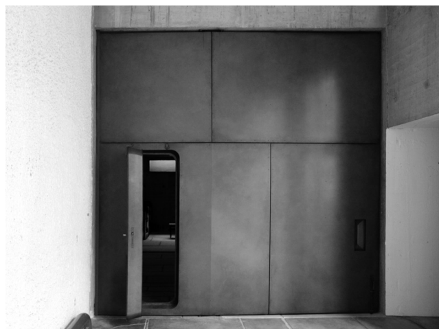
05 Le Corbusier, Couvent de La Tourette , Eveux, France, 1953-1960. South church pivot door built by Mortamet in 1989 following the unbuilt 1959 design of Le Corbusier. © FLC/SPA, ACT, Roberta Grignolo.
