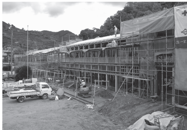
05 Matsumura Masatsune, Hizuchi Elementary School, Yawatahama, Japan, 1958. Restoration work in progress. Timber structures were strengthened to meet the earthquake resistance requirements under the current Building Standard Act. © Yoshiaki Hanada, 2008.
