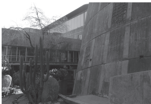
10 Emilio Dubart, ECLAC building, Santiago, Chile, 1966. Reuse design by O1ARQ, Pablo Saric, Cristian Winckler, Felipe Fritz, 2011. The new Pavilion, as seen from the base of the Caracol . © Horacio Torrent, 2014.
