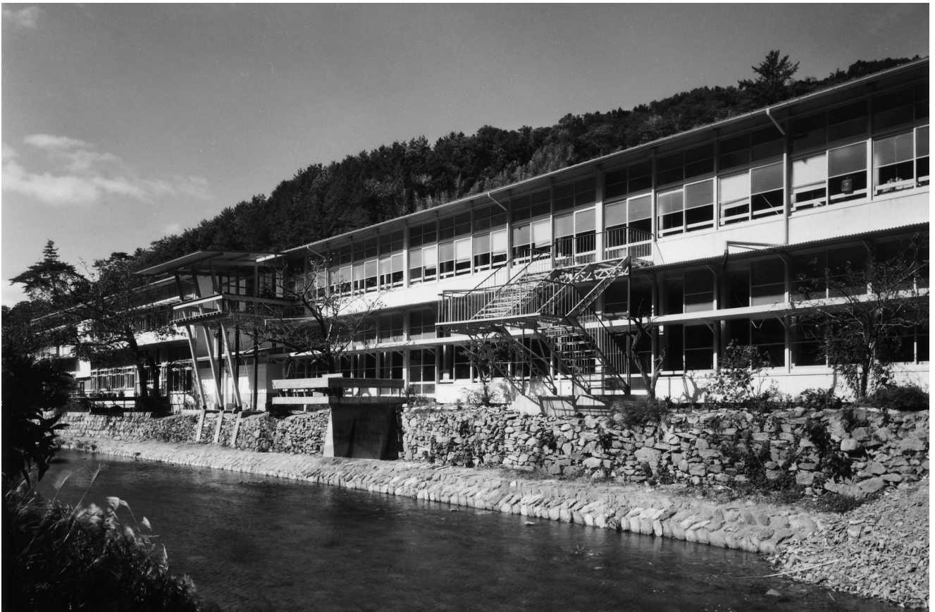
03 Matsumura Masatsure, Hizuchi Elementary School, Yawatahama, Japan, 1958. A suspended outdoor balcony and floating staircases protrude over the river. © Architectural Institute Japan Shikoku Chapter / Former property of Matsumura family, 1958.
