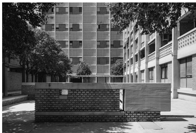
06 Santiago Artal, Santa Maria Micaela Housing . Cooperative, Valencia, Spain, 1958-1961. Presence of shuttering in circulations and terraces. © Ximo Michavila, 2007.
