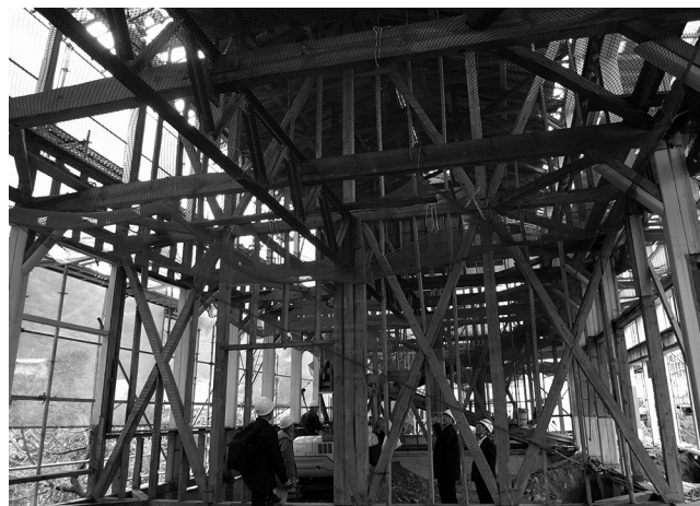
03 Restoration work in progress. © Yoshiaki Hanada, 2009.
