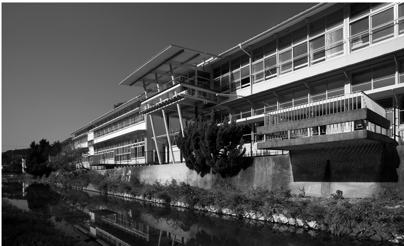
01 General view from south. © Toru Kitamura, 2009.
