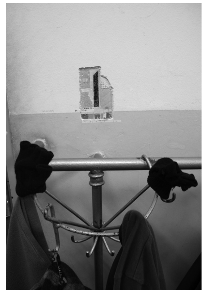
Figure 7. Original coat rack with integrated heating. Color research (2009) at the position of class number "1". © Photo by wessel de jonge architecten.
