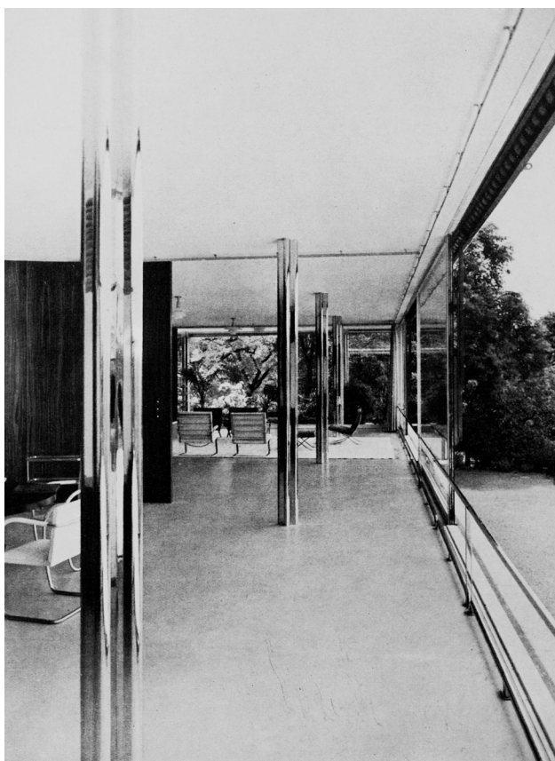
Figure 3. The chrome-plating camouflages the static function of the structure.
