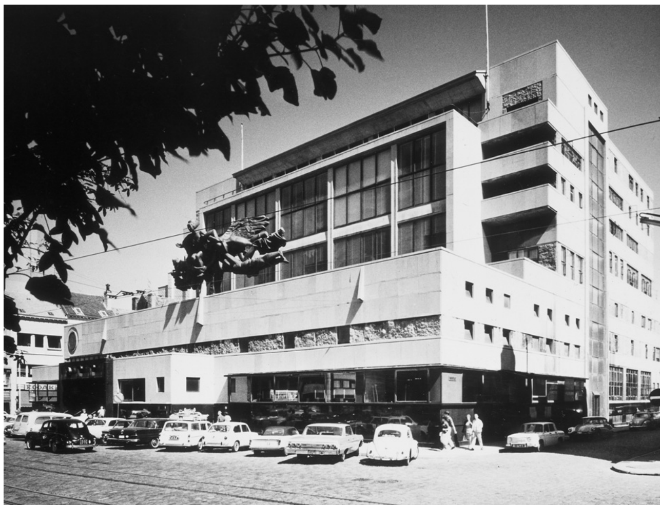
Gaston Eyselinck and his Masterpiece. The Post Office Building in Ostend (1945-1953)
