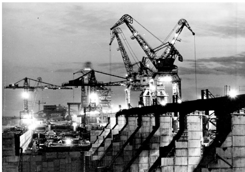
Figure 1. Kremenchug Hydroelectric Power Plant, Svetlovodsk, October 2, 1959.
