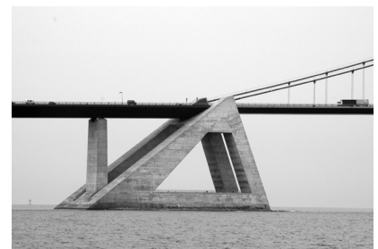
Figure 14. The East Bridge anchor block.
