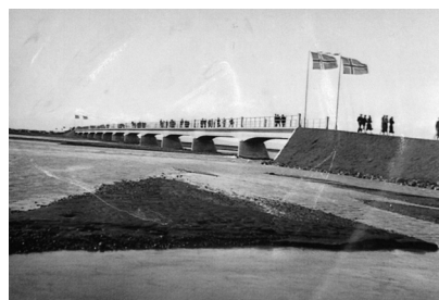
Figure 1. Restored bridge over the Fnjóská River, North-Iceland (1908). The longest span of a reinforced concrete arch in Scandinavia at the time of construction (55 m). Photo by Pétur H. Ármannsson
