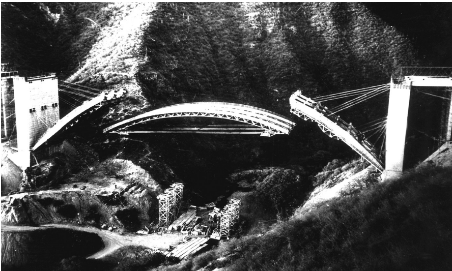
Figure 31. The middle centering ready to be lifted. The built part shows the segment webs without the upper slab.
