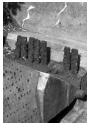
Figure 5. The end of the arch and one of the prefabricated elements before being placed.
