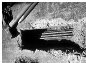
Figure 4. The prestressed bars
