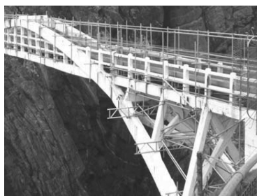
Figure 1. Temporary access scaffold supported directly from the arch ribs erected in June 2005.
