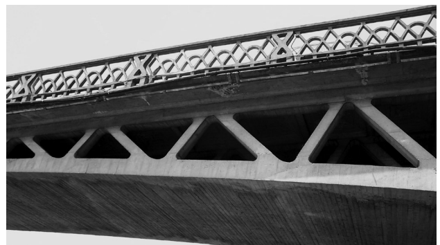
Figure 9. Detail of original railings and a concrete section of 6x6cm intact after 100 years. What a lesson!
