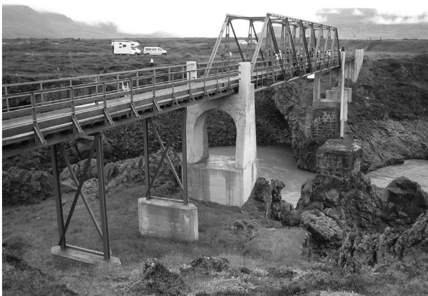
Figure 1. Restored bridge over the Fnjóská River, North-Iceland (1908). The longest span of a reinforced concrete arch in Scandinavia at the time of construction (55 m). Photo by Pétur H. Ármannsson
