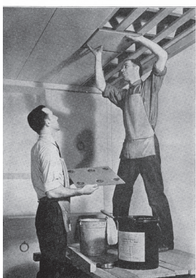
APPLICATION OF INSULATING TELEBOARD TO CEILING BY MEANS OF AN AIRBOTE Courtesy of Armstrong Cork Products Co., Lancaster, Pa.
