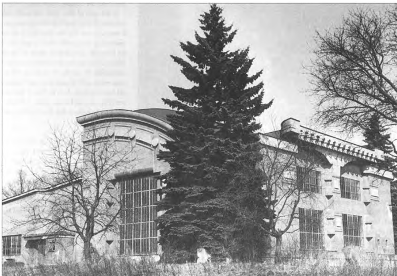
The Power Station in Háj near Mohelnice
