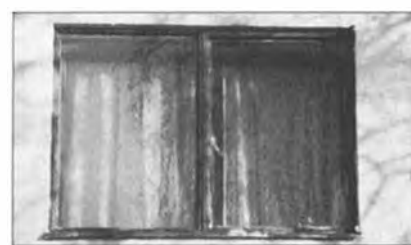
Original steel-framed window.
