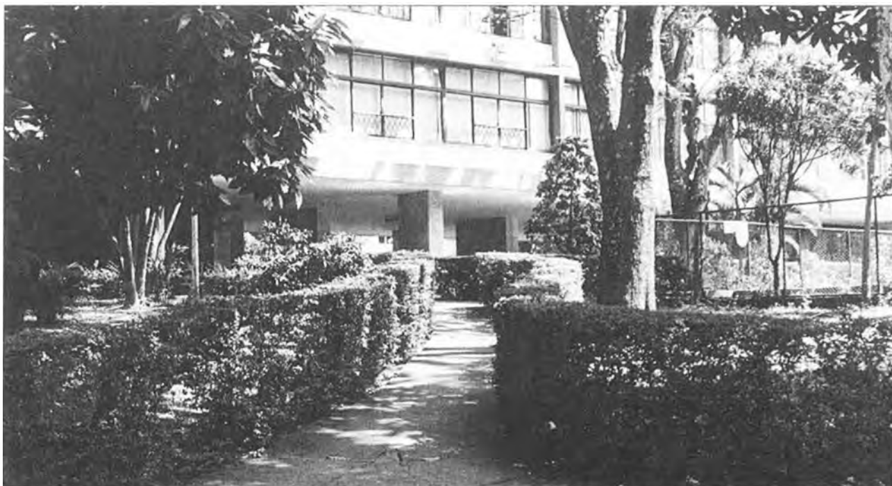
Pilotis Area: Pedestrian Access to apartment block
