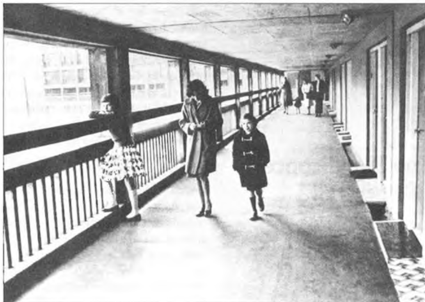
A view of the deck. Photo: Roger Mayne, for Architectural Design of September 1961
