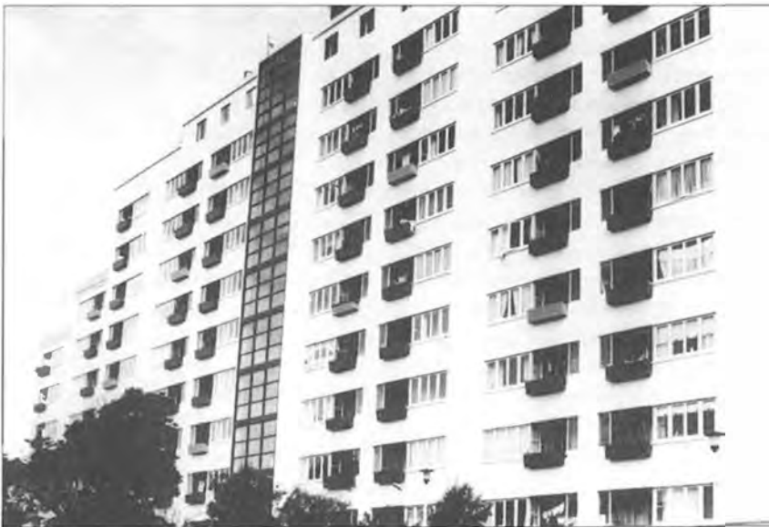
Dixon Street Flats, 1941-44, East elevator. Photographer: Julia Gailey, August 1995
