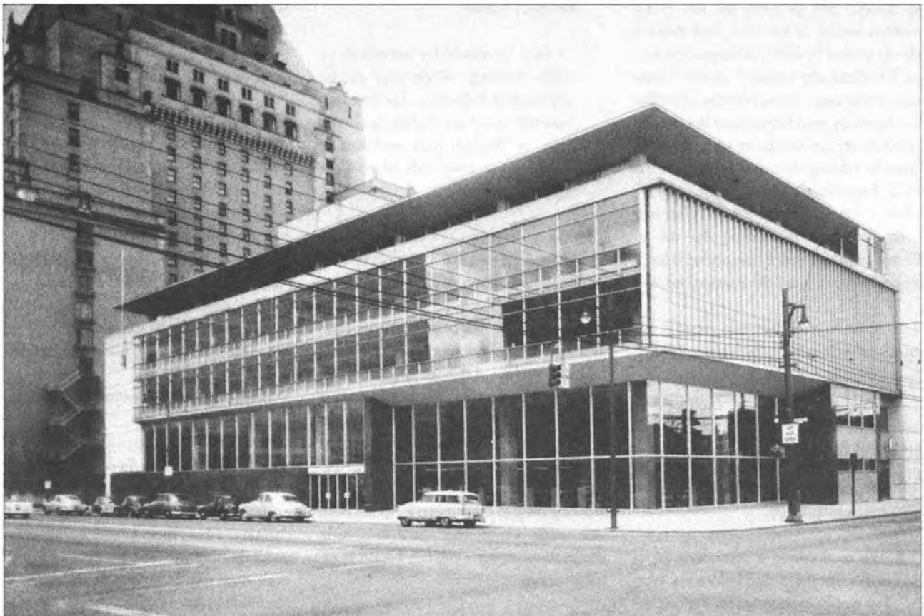
The B.C. Hydro Building was the headquarters of Vancouver's water supply company. After the refurbishment, the building serves as an apartment building. Photo: Dany Singer Photography, 1994
