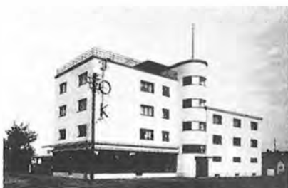
Erkki Huttunen, commercial and office building in Rauma, 1930-31.
