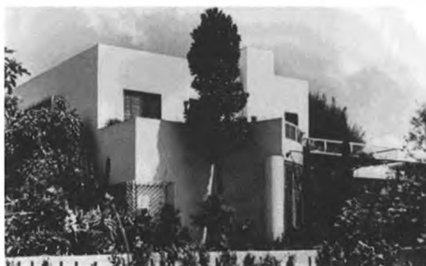
The house of 1934: the new terrace in concrete.
