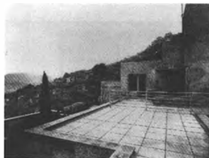
Terrace and guarding in front of the guest room on the second floor, 1928.
