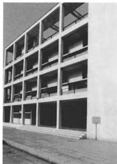
Casa del Fascio, detail of principal facade after the restoration.
