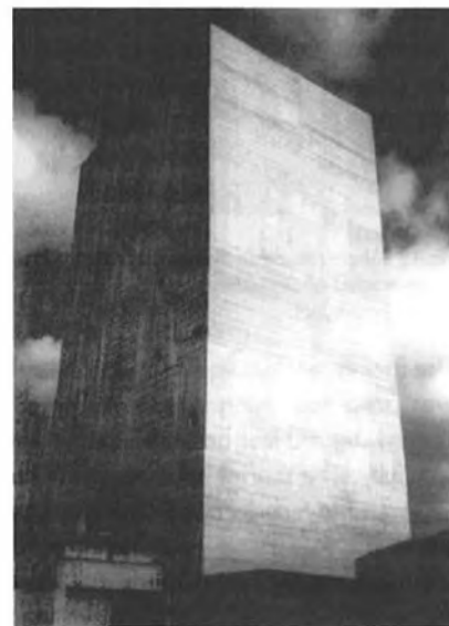
Fig. 14 The elevator turret in 1991 returned to the original appearance with the texture of the 'beton brut' and the patterns left by the wooden shuttering.
