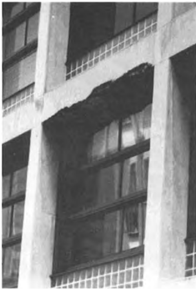
Casa del Fascio, detail of side facade before the restoration.
