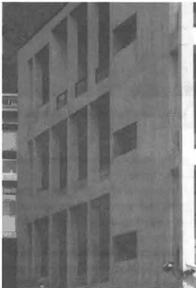
Casa del Fascio, detail of principal facade after the restoration
