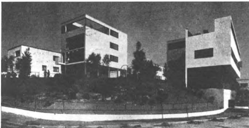
One- and two family houses in the 'Weissenhof' Werkbund Estate, architect Le Corbusier and P. Jeanneret.
