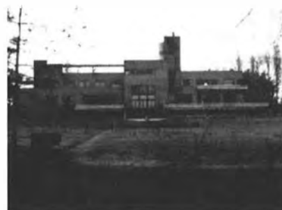
The Cavois house, the south facade, view from the park, 1989.
