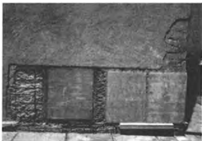
Fig.12 Samples made on the elevator turret to choose the product whose texture was most similar to that of the original.
