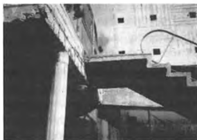
Fig. 2 - 3 General deterioration of reinforced concrete structures of the terrace.
