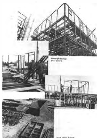
Steel framed's construction of terraced house in 'WUMA' Werkbund Estate, architect E. Lange.
