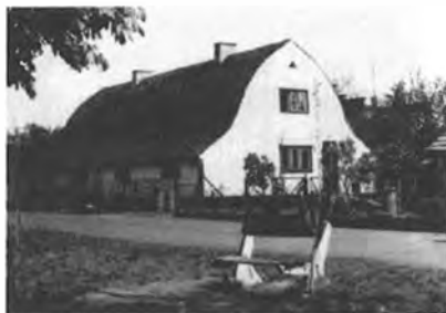
Semi-detached housing type with so-called Bohlenbinderdach.
