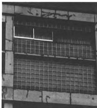
Casa del Fascio, detail of side facade before the restoration.
