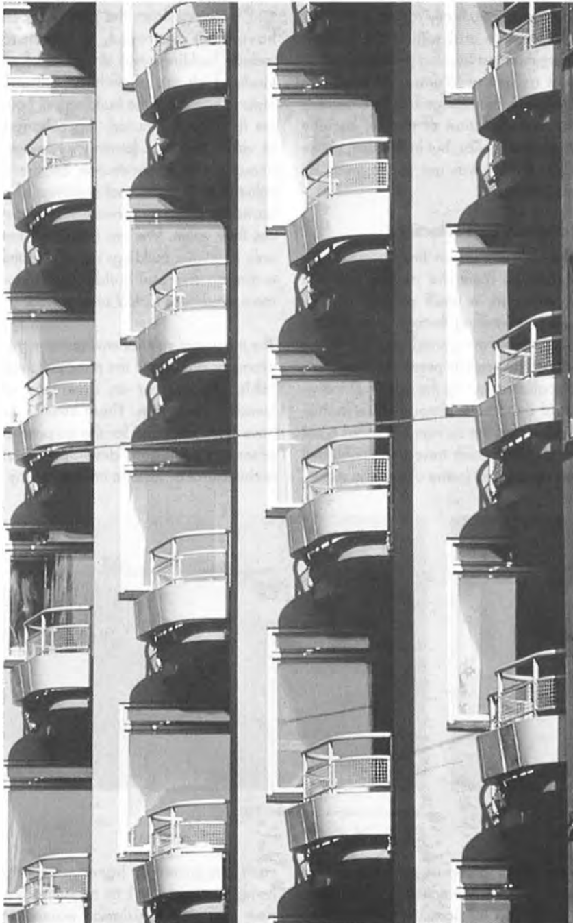
The collective house in Stockholm, architect Sven Markelius, 1935
