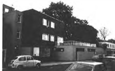
Levy House, present state.
