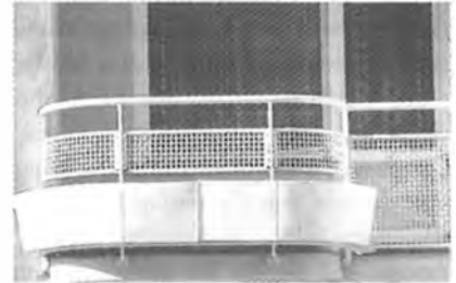
One of the balconies at the Collective House.
