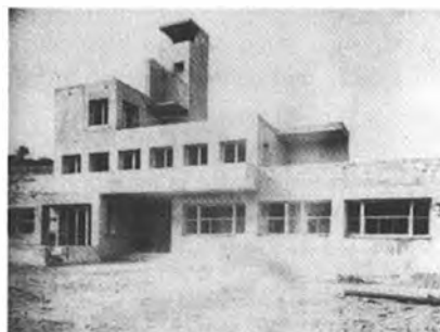
The buildingsite after instalment of the woodwork (August 1925)
