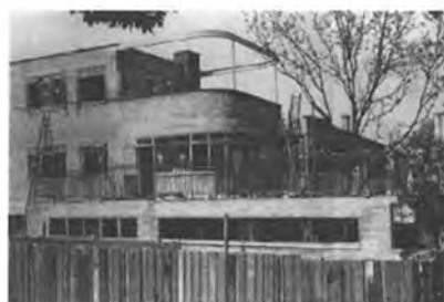
Levy House under construction, early 1936.
