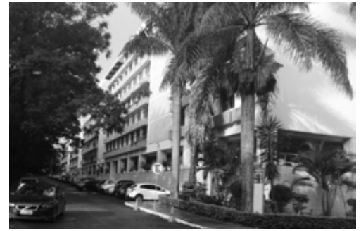
Fig. 5 Excessive landfill. Photo by Jose Galbinski
