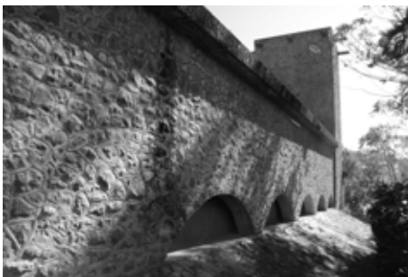
Fig. 4 Exterior, Bandarawela Chapel. Image courtesy of David Robson
