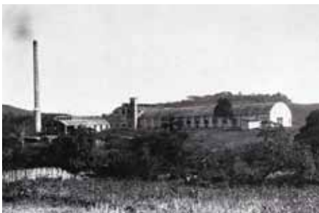
Figure 5. C&N. The Pernambuco Paper Mills Ltd. Plant. Credits: C&N files.
