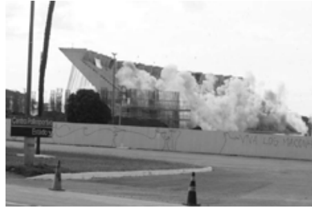
Fig. 4 Demolition of the Mané Garrincha Stadium.
