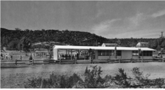
Fig. 3 CAPFCE. Elementary School in Baja California Sur. Baja California. Mexico, 1960. Memoria del CAPFCE. 1952-58
