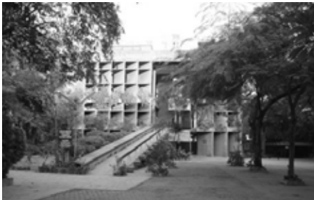
Fig. 2 Le Corbusier, the Millowners' association headquarters, Ahmedabad, India, 1951-54, west façade fins, courtesy Mr T. K. Ghoshal.
