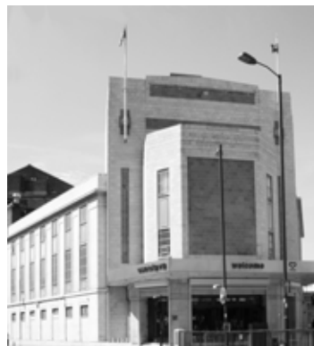
Fig. 2 E. A. Stone. Astoria , Finsbury Park, London, 1930. Main Entrance.
