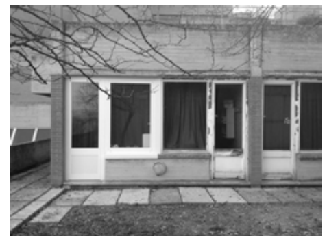
Fig. 4 Giancarlo De Carlo, Collegio della Vela, Urbino, Italy, 2014, the original timber window on the right, compared with a new PVC window. (Canziani)”
