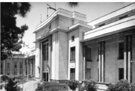
Fig. 4 Vartan Hovanesian, Central Building of Bank Sepah, Tehran, Iran, 1951
