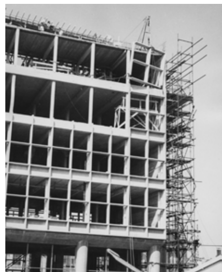
Fig. 3 C. De Geus & J.B. Ingwersen, Eerste Technische School, Amsterdam (NL), 1955, during construction, showing how large Schokbeton elements of the sun screen are hoisted in place. Photo: Jan Versnel, collection NAI Rotterdam.
