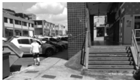
Fig. 3 Stairs & sidewalk at the end of a gallery Photo by Jose Galbinski
