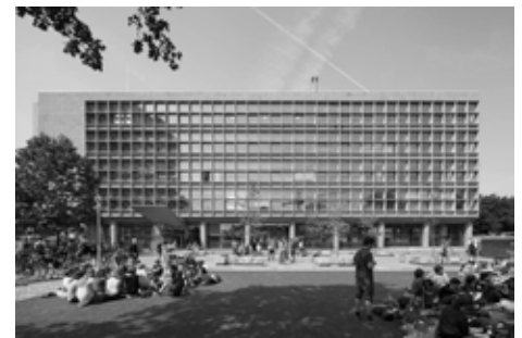
Fig. 1 C. De Geus & J.B. Ingwersen, Eerste Technische School, Amsterdam (NL), 2013, after restoration, showing the repaired Schokbeton façade panels and sunscreen elements. Photo: Raoul Suermondt
