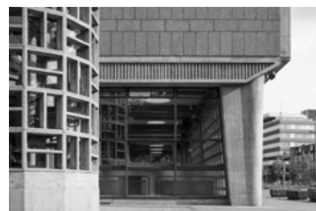
Fig. 4 C. De Geus & J.B. Ingwersen, Eerste Technische School, Amsterdam (NL), 2013, after restoration, showing the repaired Schokbeton elements of the cylindrical emergency staircase (left) and façade panels (top), and the 'chassis' on pilotis of cast-in-situ concrete. Photo: Raoul Suermondt.
