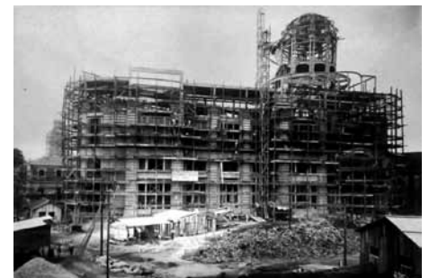
Figure 4. Hyppolito Pujol Junior, States Pavillon, Construction site and the process of building the pavillon with reinforced concrete. Credits Revista Brasileira de Engenharia.
