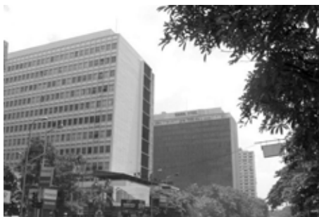
Fig. 3 Maxwell Fry, Jeevan Deep, Kolkata, India, 1957, precast panels for external shading devices, Wikimedia open source
