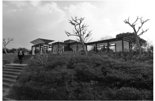
Fig. 4 Tsutsujigaoka Resthouse at the 1970 world expo in Osaka, rebuilt in 1992.
