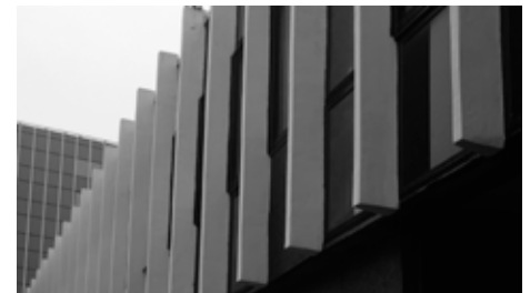
Fig. 1 Ado Eigi and Jüri Jaama, New Radio Building, Tallinn, Estonia, 1972. Original concrete ribs are still visible in the lower back wing while the highrise part has been completely renewed. Maris Mändel, 2014
