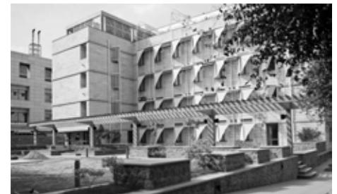
Fig. 5 Ashok B. Lall, The Institute of Rural Research and Development, Gurgaon, India, 2010, ecologically sustainable LEED Platinum rated, architect.
