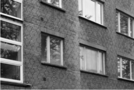
Fig. 3 House in Vase Street 4, Tallinn, Estonia, 1950s-1960s. Use of elaborate decorative brick bond was unusual in a Soviet context. Maris Mändel, 2014
