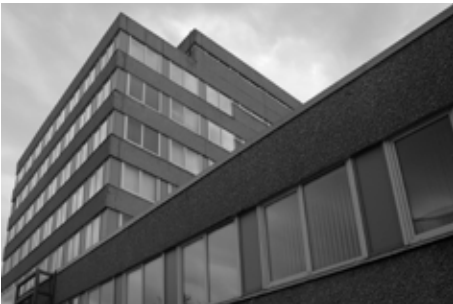
Fig. 4 Administrative building of Ilmarine Plant, 1975-76. Specially designed decorative oil shale ash concrete panels with gravel coating. Maris Mändel, 2014
