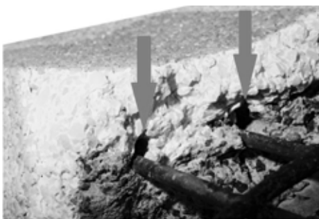
Fig. 5 MLC Centre Tower
