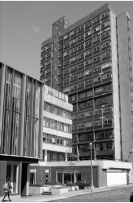
Fig. 1 Robert Matthew, Johnson-Marshall & Partners, Adam Ferguson Building, Edinburgh, Scotland, 1965-67, South Elevation - new extension and infill of plinth. Caroline Engel
