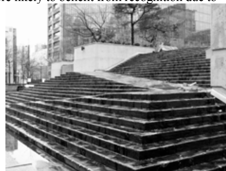
Fig. 5 Arthur Erickson with C.H. Oberlander, Robson Square Law Courts, Vancouver, Canada, 1973-1983. Installation of new roofing membrane at "stramps," part of Robson Square renewal by Omicron, 2009. J. Ashby.
