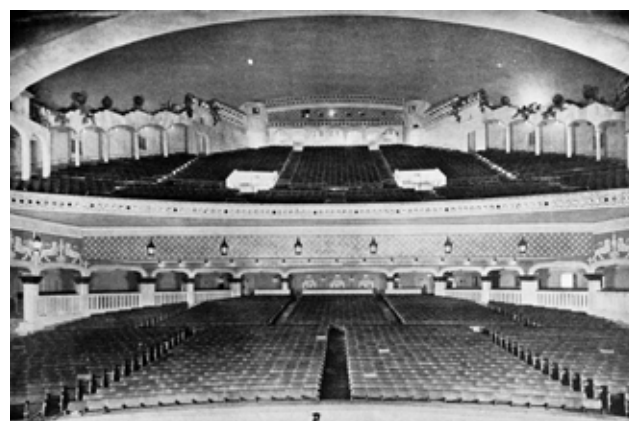
Fig. 5 E. A. Stone. Astoria, Finsbury Park, London, 1930. View of the auditorium from the stage. (Source: The Builder , vol. 139, 563-568).
