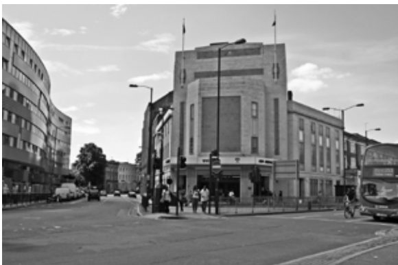
Fig. 1 E. A. Stone. Astoria , Finsbury Park, London, 1930. Main Entrance.
