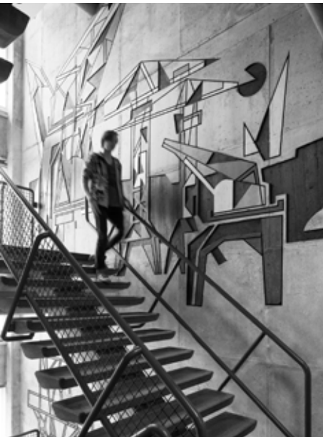
Fig. 6 De Geus & J.B. Ingwersen, Eerste Technische School, Amsterdam (NL), 2013, main staircase with Schokbeton stairs and the principle bas relief by the artist Harry op de Laak, after removing the peach-coloured paint from the concrete wall by snow blasting. Photo: Raoul Suermondt.
