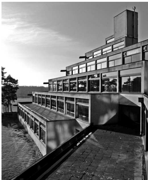
Figure 1. UEA: Ziggurats of residences by Denys Lasdun & Partners, 1965-67. Photo: CAR.
