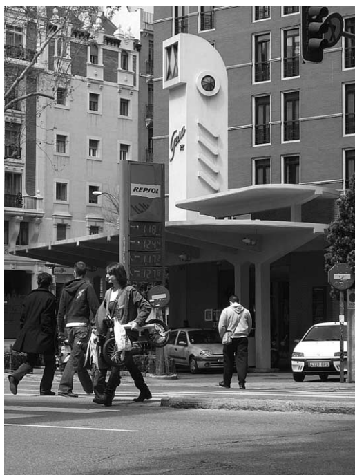
Figure 2. The reconstructed building in 2008. Photo: David Rivera Gámez.
