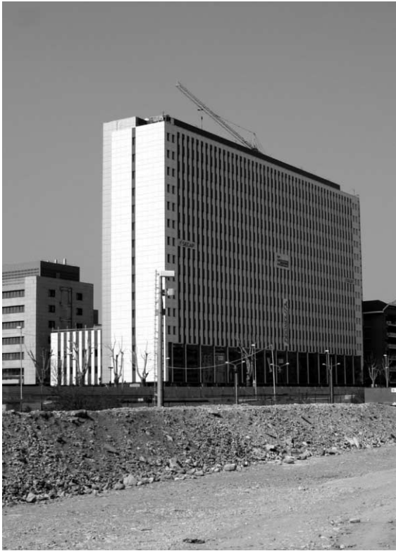
Figure 2. The design of façade after the renewal, April 2008. Photo: Fabio Sarcone.
