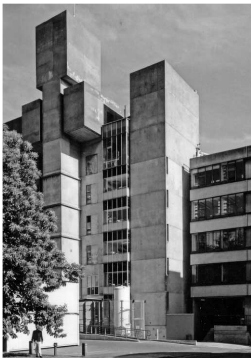
Figure 2. UEA: Teaching Wall by Denys Lasdun & Partners, 1964-74. Photo: CAR.
