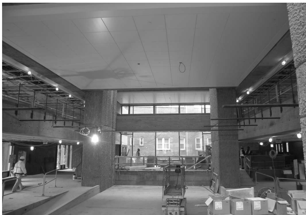
Figure 2. A&A Building, renovation progress, 2008. Photograph: Nina Rappaport.
