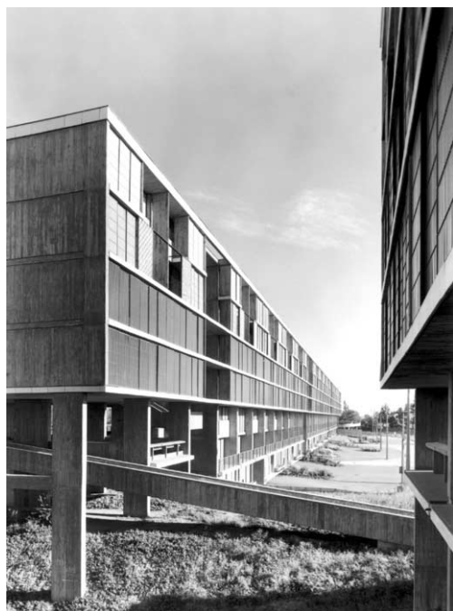
Figure 1. Exterior view of Block n° 1.
