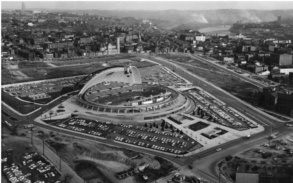
Figure 3. View of Arena Roof in open position, circa 1961. Provided by the architect's successor firm Deeter Ritchey Sippel.
