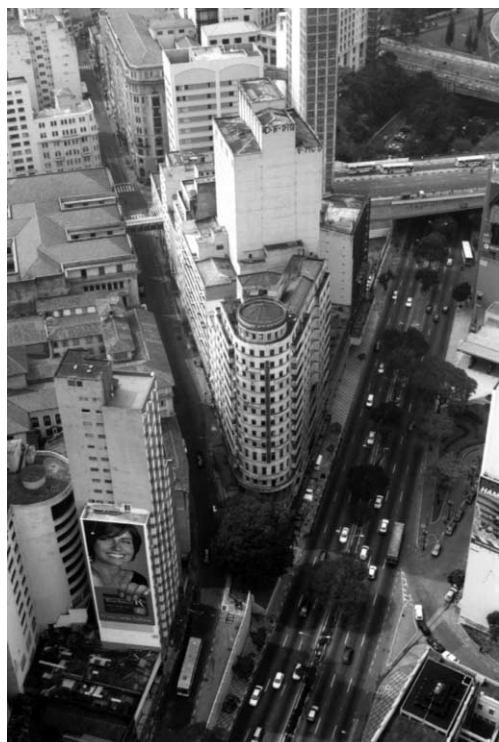
Figure 3. Aerial view of the building, before the rehabilitation. Photo: COHAB-SP.
