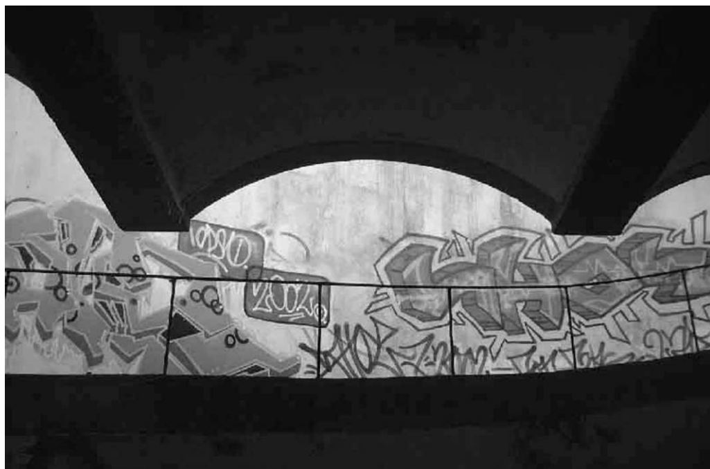
Figure 2. Cardross Seminary: condition in 2007. Architects Gillespie, Kidd and Coia. Photograph: authors.
