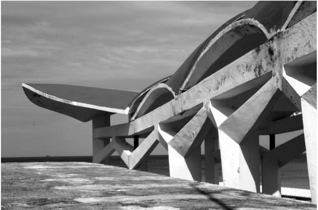
Figure 2. Detail of the vaulted entrance to the resort, the lobster. Photo: Isabella Fera
