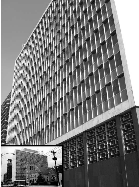
Figure 2. 615 Peachtree Building (former First National Bank Building), constructed 1958, demolished 2006. Smith & Smith, architects, Atlanta, Georgia. Image by author, inset 1960 photo from Georgia State University Archives.
