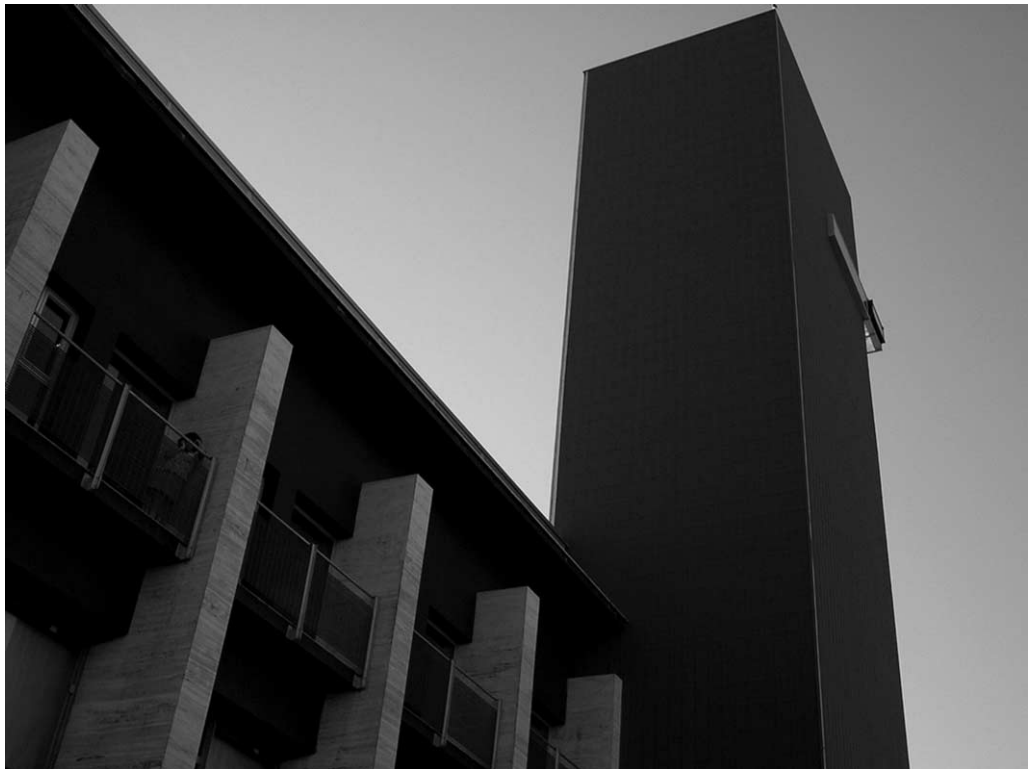
Figure 4. A modern layout dressed in new materials. Photographer: Pablo Oliver.
