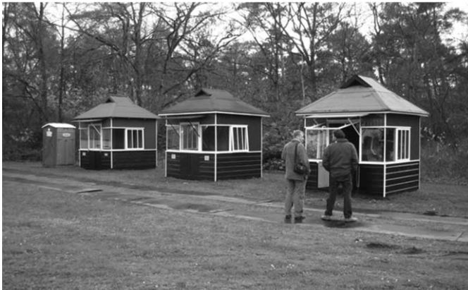
Figure 2. Three restored boshuisjes in row, November 2007. Photo: W. Bulten, private archive, Delft.
