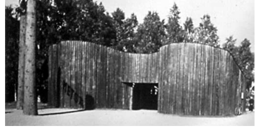
Figure 3. Photography of Lapua Pavilion, 1937. Source AAA.
