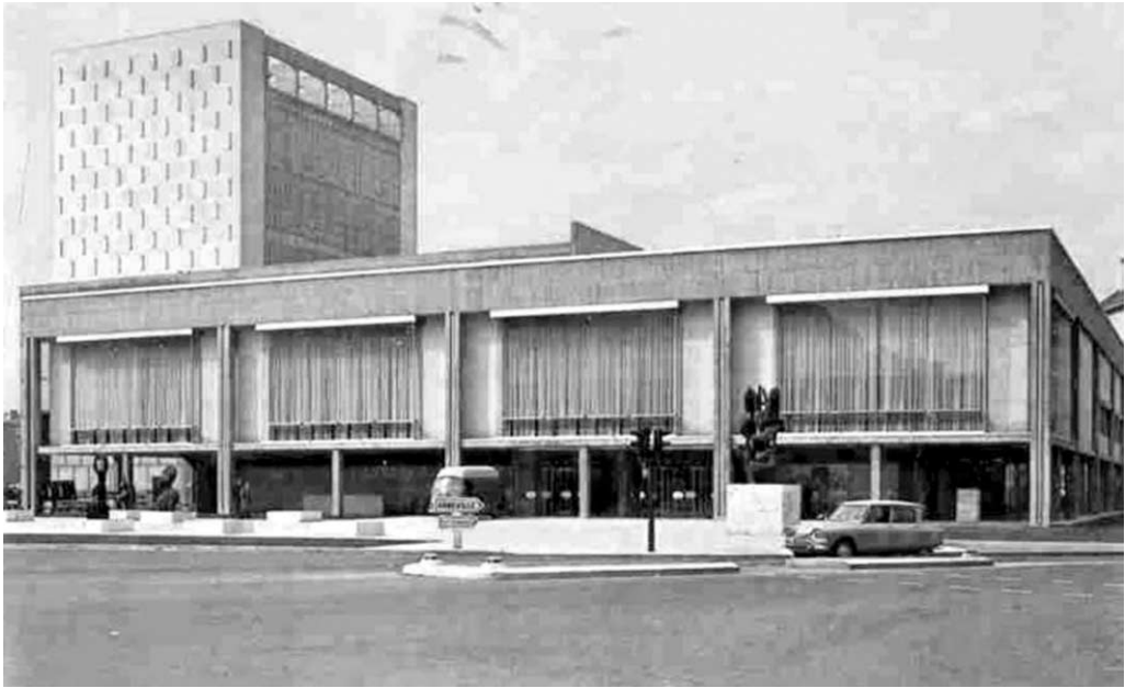
Figure 2. Maison de la culture in Amiens (1961-1965) Pierre Sonrel, Jean Duthilleul and Marcel Gogois architects, old postcard.
