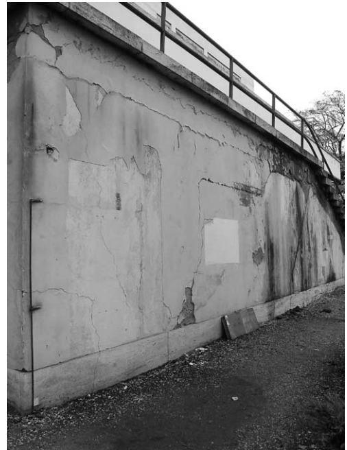
Figure 4. Brno, Tugendhat House, garden staircase, paint containing water impermeable resin (2003).
