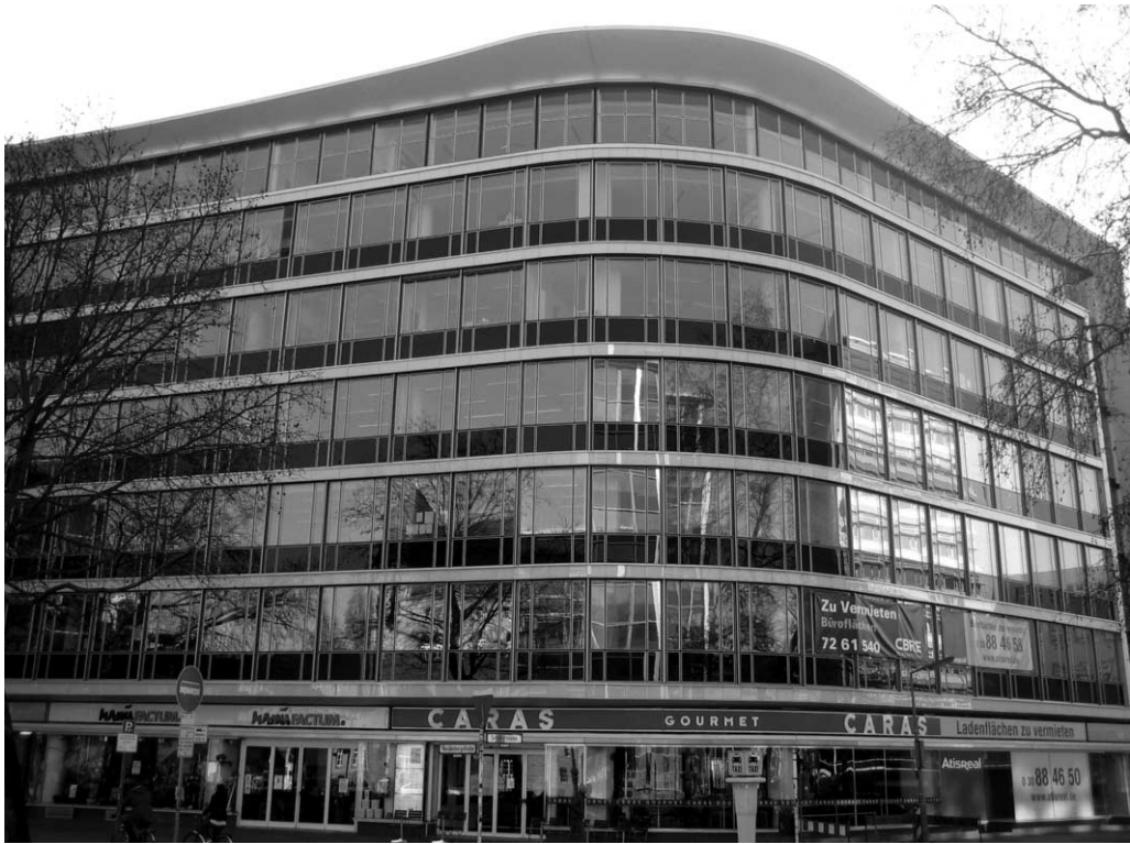
Figure 1. The original steel facade of Haus Hardenberg in Berlin from 1956 has been completely restored in 2004. Photo: author.
