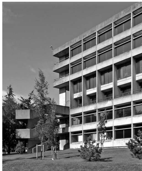
Figure 3. UEA: Library by Denys Lasdun & Partners, 1965-74. Photo: CAR.
