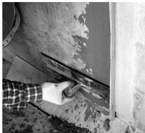
Figure 4. In situ mock up of repair materials being conducted. Photo: Amanda Thomas Trienens, copyright: Solomon R. Guggenheim Museum.
