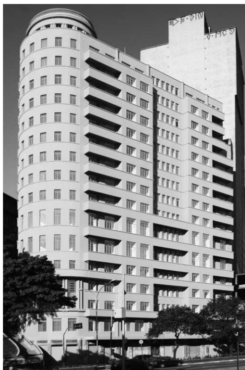
Figure 4. West façade of the building, after the rehabilitation. Photo: Sonia Gouveia.
