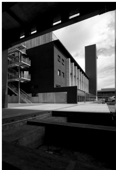
Figure 2. The re-used Concepción railway station among the new structures. Photographer: Cristóbal Palma.
