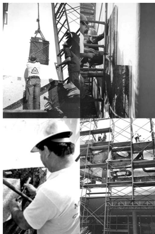
Figure 4. Mechanical Anchor System of Veneer panels applied during the restoration of "Amelia Peláez Mural". Habana Libre Hotel, 1998.
