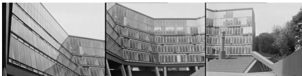
Figure 2. Stills showing u-shaped interior of the Florey building from Jim Stirling's Architecture , Directed by Ron Parks, 1973. Copyright holder is Arts Council England.
