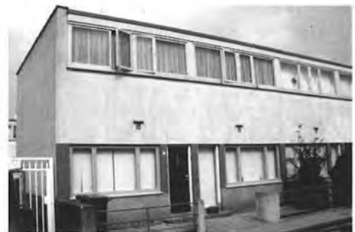
Rotterdam, Kiefoek housing estate, a row of the reconstructed houses showing the internal junction by means of a large glass opening instead of a door (Photo by Marieke Kuipers, 2001).
