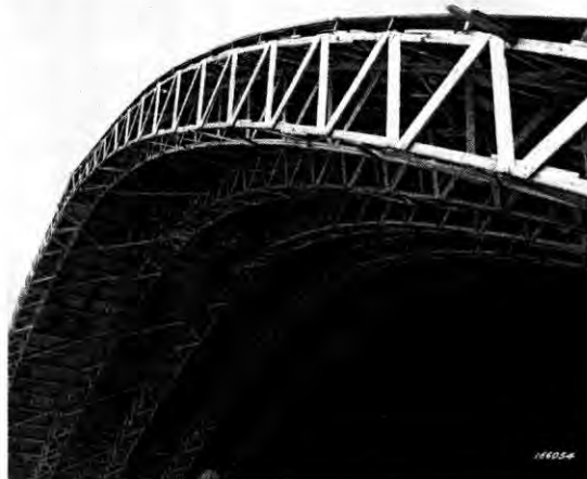
Fig. 5 – Construction of bows of repair hangar 46 hangar at an Engineer installation at 4th Air Depot, Townsville, Australia December 1942 Photograph: Pvt Joseph Herda. Signal Corps Photo #GHQ-SWPA-SC-43-2418-195-147E/SC166054. Held National Archives and Records Administration, College Park, Maryland, USA.
