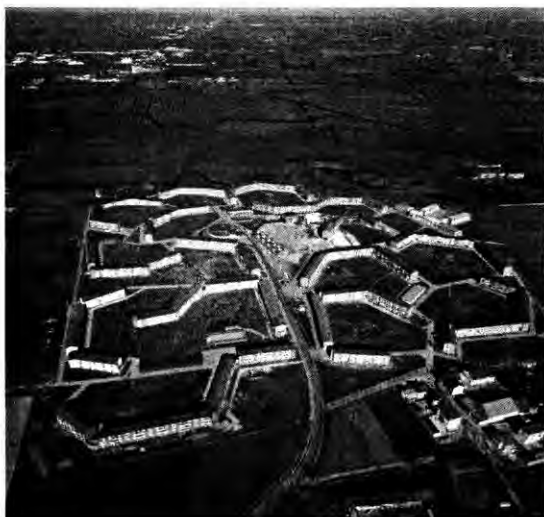
Fig. A2 – Aerial View
