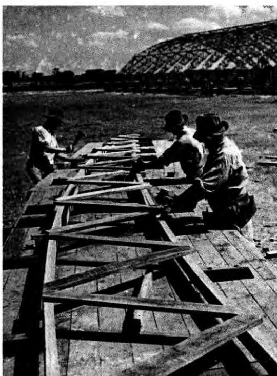
Fig. 2 – Carpenters pre-fabricating bow-truss cord [sic] on specially constructed table. Rydlemere. Construction US Stores. February 1943. Item 53.1/2.4, box 17, series B5281, National Archives of Australia.
