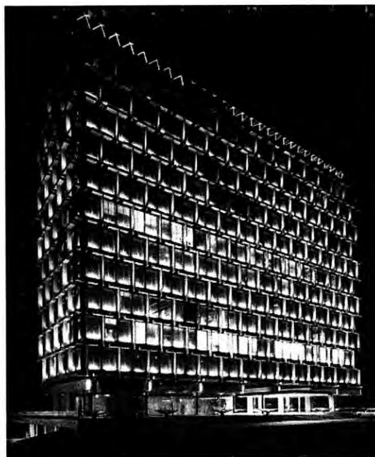
Fig. 2 – Entrance foyer of Council House illuminated at night, Richard Waldendorp, 1963.
