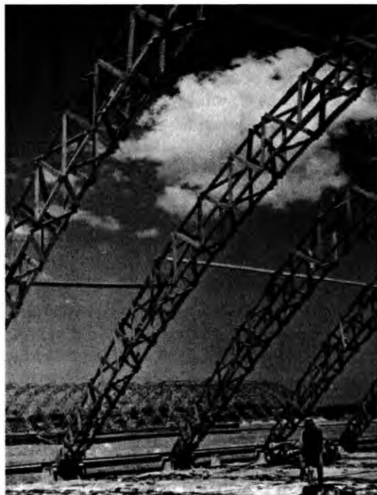
Fig. 3 – View of walls, abutment pads and arches. 2nd store in similar stage of construction. Rydlemere. Construction US Stores. February 1943. Item 53.1/2.7, box 17, series B5281, National Archives of Australia.
