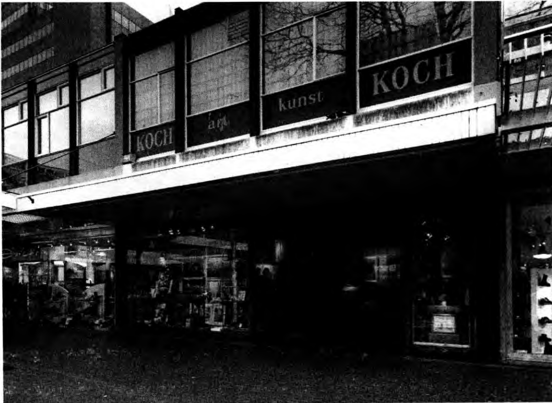
Fig. 6 – Front of Koch's art shop, the only remaining authentic element of the original layout of the Lijnbaan. Photo: RDMZ, Zeist, 1999.
