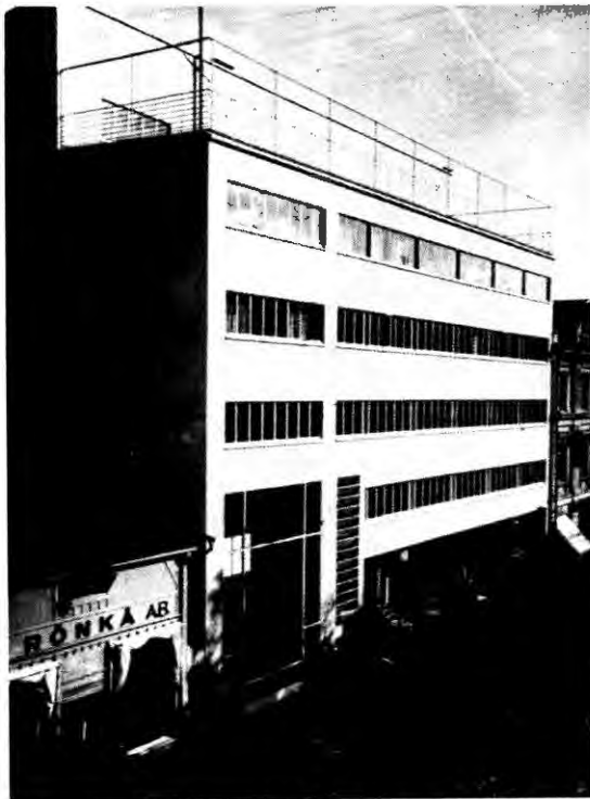
Fig. 1 – Alvar Aalto, building of the Turun Sanomat, Turku (Finland), 1929 (Photograph G. Welin, Museum of Finnish Architecture)
