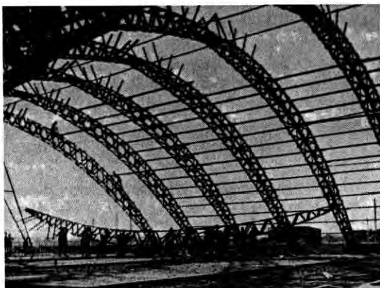
Fig. 7 – Members of the [Civil Construction Corps] mobile unit wheeling prefabricated bow trusses into position for erection. Townsville – Gorbett – RAAF Store. July 1943. Item 53.3/1.4, box 1B, series B5281, National Archives of Australia.
