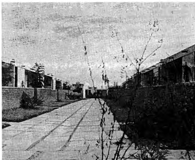
Fig. 12 – A street and houses in a 5th degree community in Islamabad. Source: Daxiadis archive.
