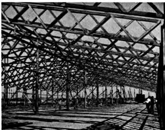
Fig. 1 – Erection of prefabricated framework. Three hundred feet of roof trusses were erected in six days by 12 men. Meeandah – Warehouse construction. July 1943. Item 53.3/3.4, box 18, series B5281, National Archives of Australia.
