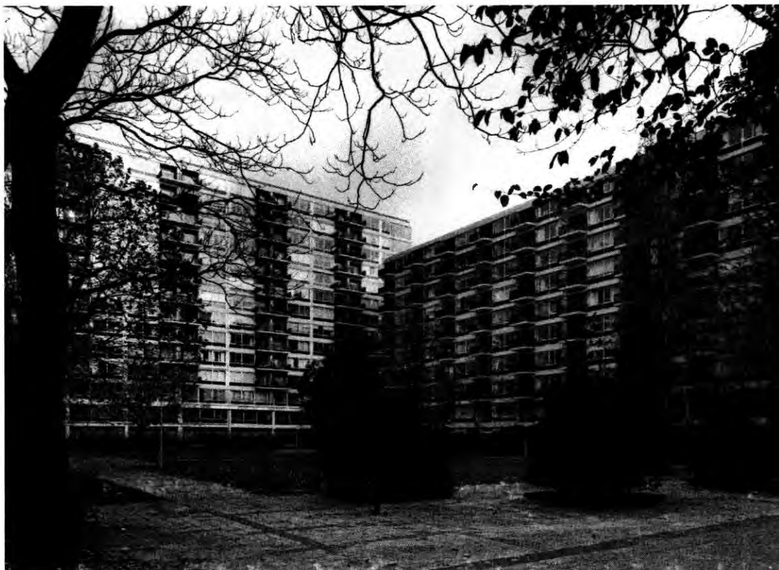
Fig. 12 – Rotterdam, Lijnbaan flatblocks with green square still functioning according to the original intentions. Photo: RDMZ, Zeist, 1999.
