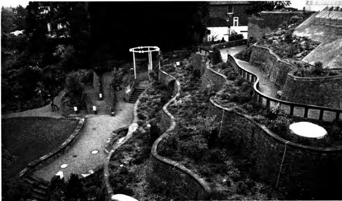
Fig. 8 – H.Hollein, Abeitberg Museum, Mönchengladbach 1972-1982. View of the garden superimposed to the roof of the museum
