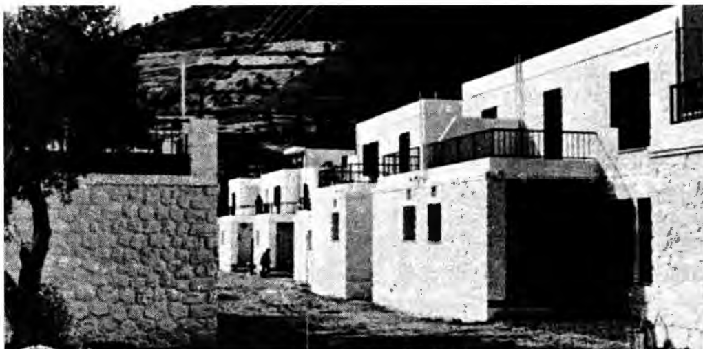
Fig. 16 – Aspra Spitia. Two-storey houses. Source: Doxiadis Associates, Aspra Spitia: A new 'Greek' city [p. 4].
