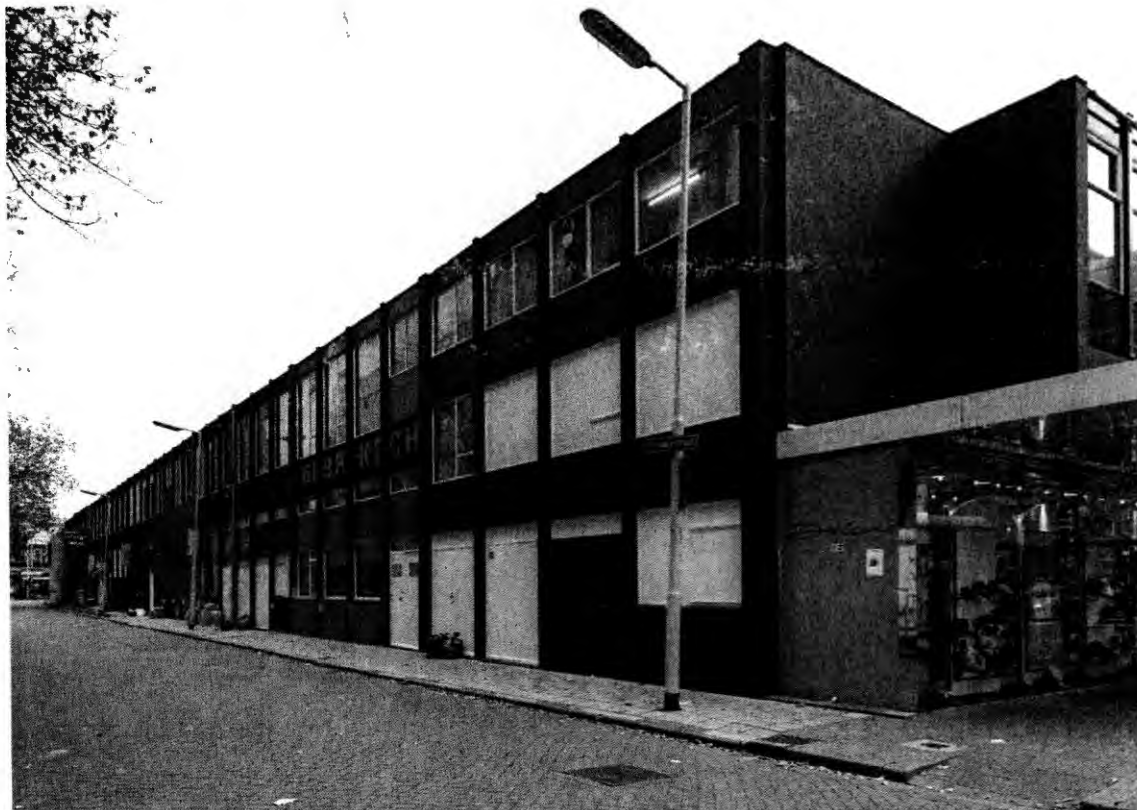
Fig. 7 – Rear of Koch's art shop and adjacent shops along the expedition street. Photo: RDMZ, Zeist, 1999.
