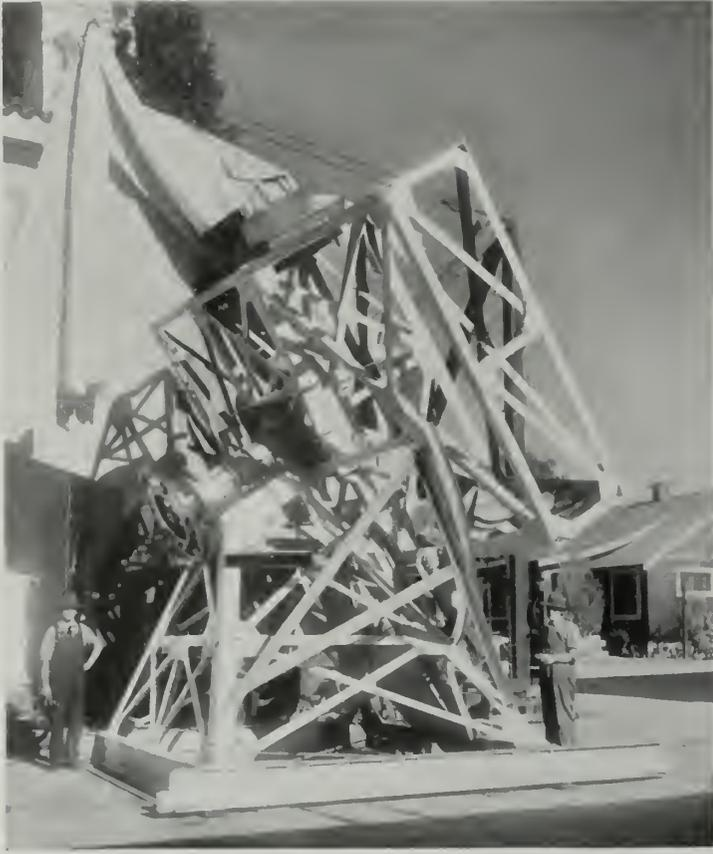
THIS MOUNTING, TO BE USED AT THE MT. WILSON STATION ON POINT LOMA, WAS DESIGNED BY MR. HALE FOR USE WITH THE NEW INTERFEROMETER ON MT. WILSON. IT WILL HAVE ATTACHED TO IT TEN OR TWELVE INSTRUMENTS DURING THE TIME OF THE ECLIPSE
