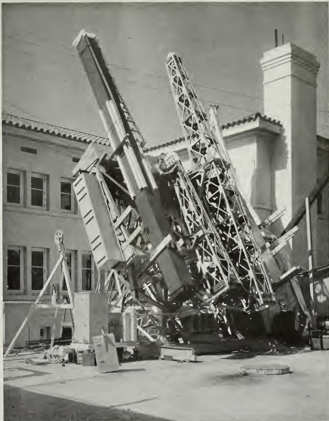
HERE THE MOUNTING SHOWN IN THIS MAGAZINE IN AUGUST HAS BEEN COVERED WITH THE TELESCOPES TO BE USED BY THE MOUNT WILSON ASTRONOMERS AT POINT LOMA DURING THE ECLIPSE ON SEPTEMBER 10. THE GREAT CAMERAS WERE PUT IN PLACE IN THIS POSITION BEHIND THE LIBRARY ON SANTA BARBARA STREET, PASADENA, AND HAVE NOW BEEN DISMANTLED AND SHIPPED TO POINT LOMA.
