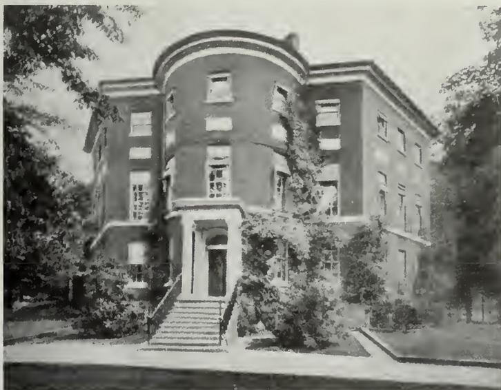
The material is red brick with trimmings of Aquia Creek sand stone.
