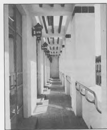
Second-floor corridor, Goldsmith Hall.
