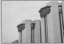
M. D. Anderson Hospital. R. Lee Clark Clinic, Pierce Goodwin Alexander, 1987. M. D. Anderson was the first TMC member to break with the style guidelines in the 1950s. The firm of MacKie and Kannah (which was responsible for several buildings at the Medical Center, including the City of Houston Department of Public Health) designed in the manner of Frank Lloyd Wright the successive stages of the hospital, first using characteristic pink marble and long sun shades, then in 1976 adding the polygonal towers and cantilevered nests of the Lutheran Pavilion. The Clark Clinic is an uninspired box.
