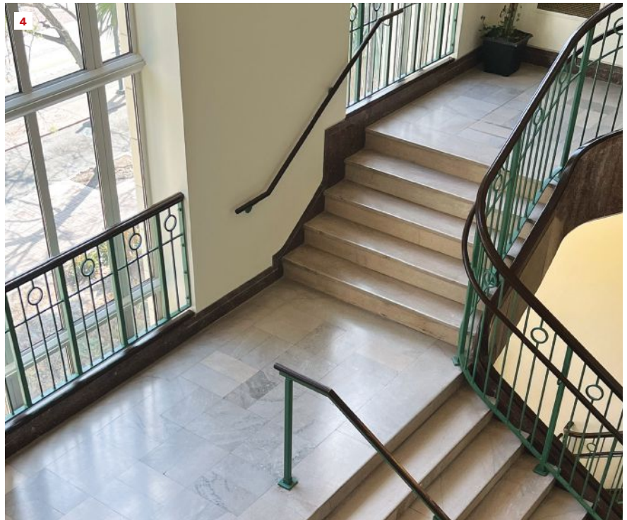
This landing (4) at the Orange County Regional History Center in Orlando, Fla., has an elongated landing that projects one tread depth beyond the line of the handrail. This unstacks the stacked risers that would otherwise occur if the corner of the landing came to a point directly below the guardrail.
