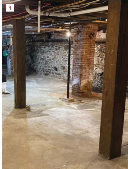
The basement before repairs (1) shows the original timber support posts holding up the main beam. A closeup of one of the basement columns (2) shows significant decay where the wood was encased in the thin concrete floor slab.
