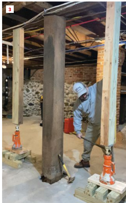
With house jacks supported on cribbing, the author began raising the jacks to take the weight off the old columns (3). To free the posts, he cut through the slab and excavated around the posts prior to raising the jacks (4). Once the old column was loose, he stopped jacking.
