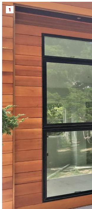
The author devised two different corner treatments using copper flashing that he has since used on a number of exteriors—an open square corner (1) and a single fin (2).
