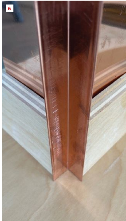
Instead of the usual decorative trim pieces that are applied after the siding is installed, these treatments are integrated into the siding during installation. These detail photos of the open square corner treatments (5, 6) demonstrate how they are installed.
