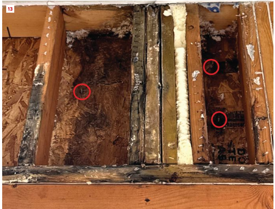
Deterioration of the OSB sheathing (12) was discovered where brick tie fasteners (circled in red) penetrated the sheathing, instead of being driven into framing (13). An infrared image (14) highlights moist areas in darker colors where water has run down the wall cavities and started to deteriorate the bottom wall plates.
