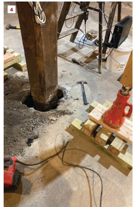
With house jacks supported on cribbing, the author began raising the jacks to take the weight off the old columns (3). To free the posts, he cut through the slab and excavated around the posts prior to raising the jacks (4). Once the old column was loose, he stopped jacking.
