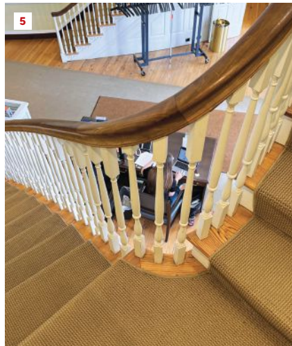
Thomas Jefferson designed this elegant stairway for his Rotunda at the University of Virginia. Rather than coming to a point beneath the handrail, the edge of the oversized, pie-shaped landing below the handrail has the same width as each tread. This unstacks the risers and allows for a smooth handrail at a consistent height above the landing and treads.
