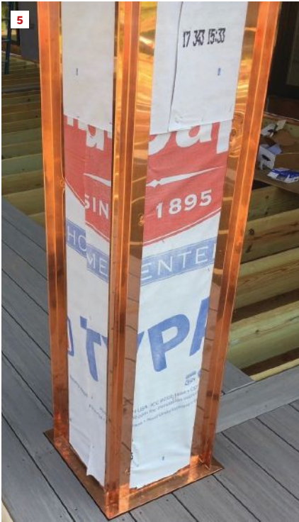
Instead of the usual decorative trim pieces that are applied after the siding is installed, these treatments are integrated into the siding during installation. These detail photos of the open square corner treatments (5, 6) demonstrate how they are installed.
