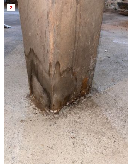
The basement before repairs (1) shows the original timber support posts holding up the main beam. A closeup of one of the basement columns (2) shows significant decay where the wood was encased in the thin concrete floor slab.
