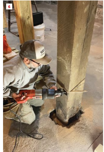
Using a straightedge screwed to the column, the author made an initial cut through the column with a circular saw (5). Following the kerf line he made with the circular saw, he finished the square cut with a recip saw (6).
