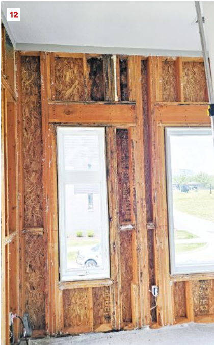
Deterioration of the OSB sheathing (12) was discovered where brick tie fasteners (circled in red) penetrated the sheathing, instead of being driven into framing (13). An infrared image (14) highlights moist areas in darker colors where water has run down the wall cavities and started to deteriorate the bottom wall plates.
