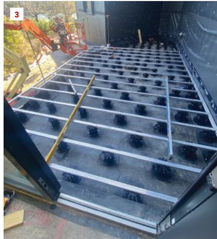
Code required a scupper in the curb opposite the center drain (2). The pedestals and rails are set so the decking will be flush at door openings (3). Note the cylindrical spacers (4) at the base of the post rods to support each post when the rods are tightened down.
