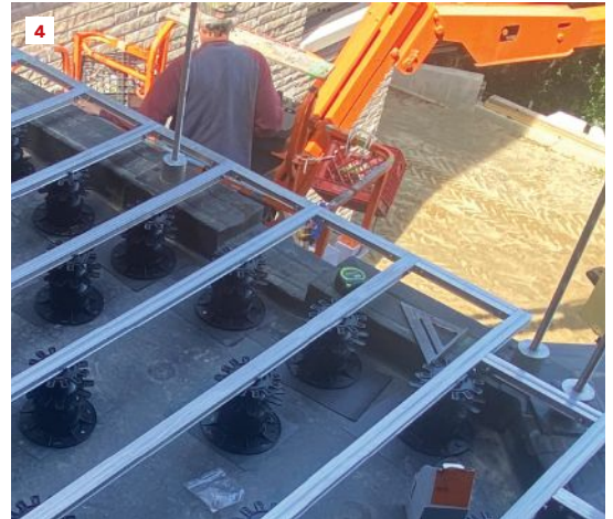
Code required a scupper in the curb opposite the center drain (2). The pedestals and rails are set so the decking will be flush at door openings (3). Note the cylindrical spacers (4) at the base of the post rods to support each post when the rods are tightened down.
