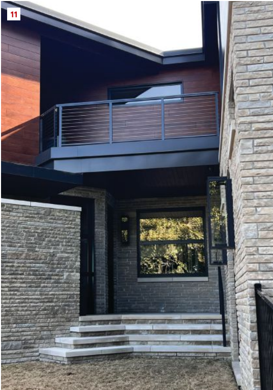
A view of one exterior porch shows the finished railing and clad fascia.
