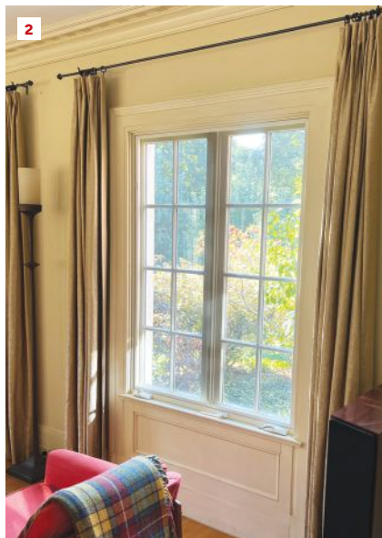
Two examples from a Classical Revival home: In its simplest form, the stool overlaps onto picture-frame trim (left). In the home's formal living areas where windows are larger, the casings come all the way down to the floor and the area below is filled-in with panels. The stiles and rails around the panels are on the same plane as the casing.
