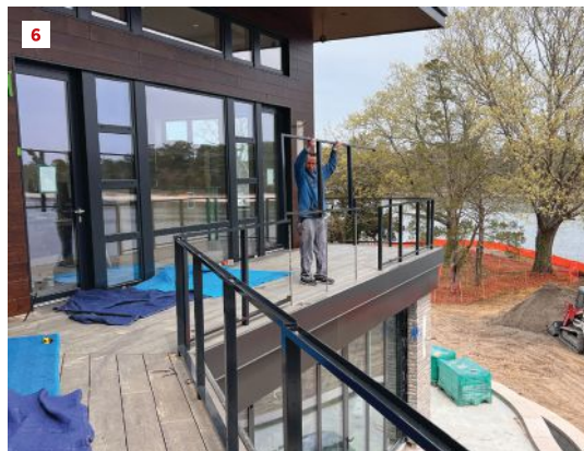
Composite decking was installed over the guard post rods (5) before the railing contractor slid aluminum railing sections over the rods (6). Once the nut on each rod is tightened down, a graspable top rail and cable completes the guard rail (7).
