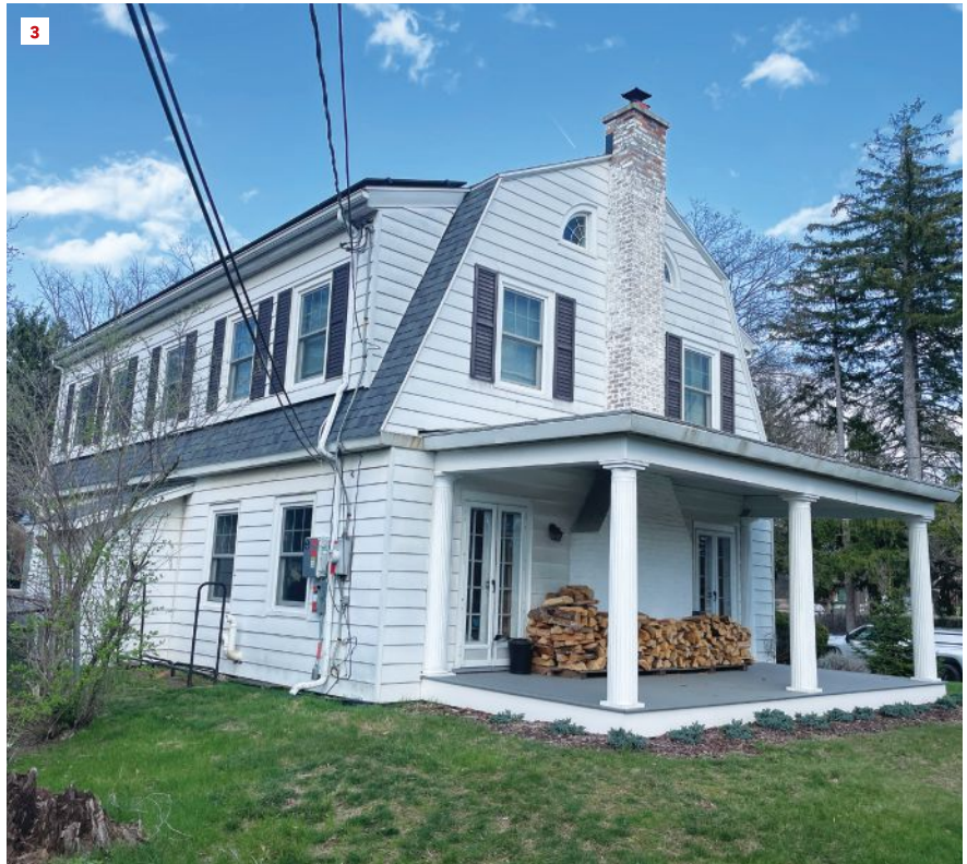
New architectural-grade shingles, a ridge vent, and a rework of the soffit venting was an important and early upgrade to the Waverly house. This scope of work included rolled SBS to replace the flat-lock tin on the side porches.
