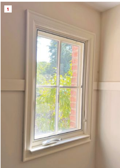
Two examples from a Classical Revival home: In its simplest form, the stool overlaps onto picture-frame trim (left). In the home's formal living areas where windows are larger, the casings come all the way down to the floor and the area below is filled-in with panels. The stiles and rails around the panels are on the same plane as the casing.
