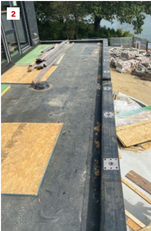
Code required a scupper in the curb opposite the center drain (2). The pedestals and rails are set so the decking will be flush at door openings (3). Note the cylindrical spacers (4) at the base of the post rods to support each post when the rods are tightened down.
