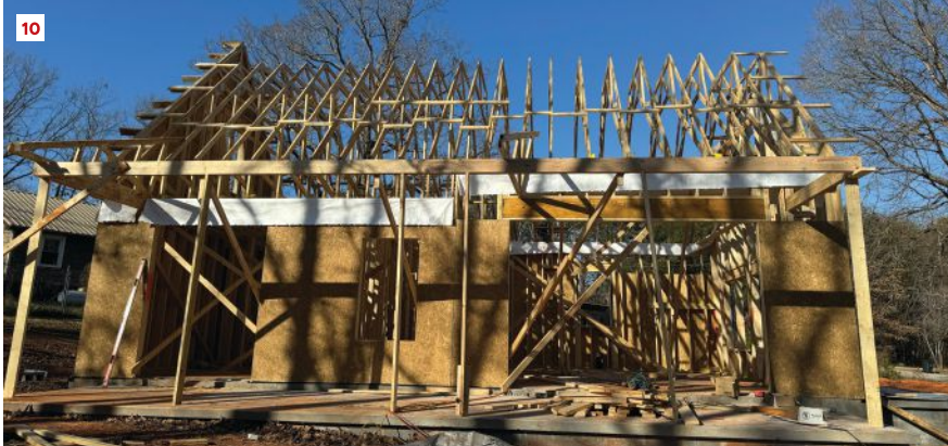
Scissors trusses over the great room (to the right) bear on 10-foot walls. The bonus trusses (on the left) sit on 9-foot walls.
