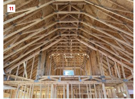
The “bonus” trusses have a parallel-chord floor structure where mechanicals will run.
