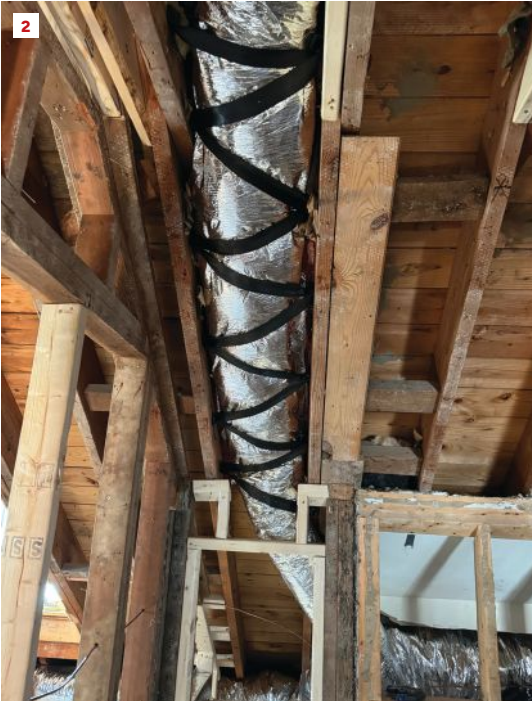
This flex duct (2) filled the whole cavity, leaving no room for condensation-controlling insulation above the duct and little room to install any insulation in the bay. The author's HVAC partner switched it out for a section of metal duct (3). That made it possible to apply closed-cell spray foam between the duct and the sheathing and to fill the cavity, which provided condensation control on the duct.
