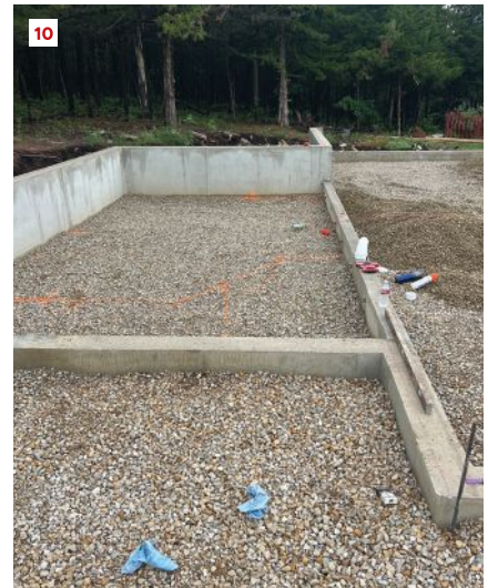
Conventional crushed stone was used for the remainder of the foundation fill (9, 10).
