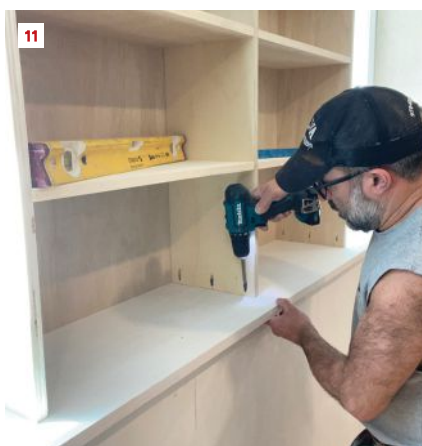
All parts are sanded before assembly moves inside (7). Shelf width is confirmed before final cut (8). Parts are predrilled to ensure alignment and to prevent screw blowout (9, 10). The units fasten to both the ledge and the wall for stability (11, 12).
