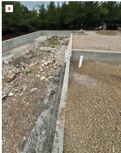
Conventional crushed stone was used for the remainder of the foundation fill (9, 10).
