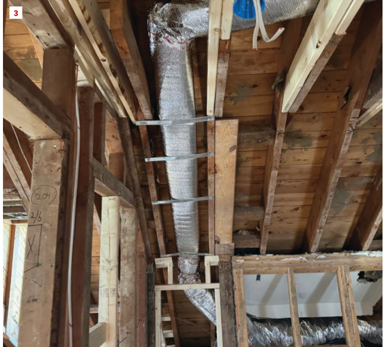
This flex duct (2) filled the whole cavity, leaving no room for condensation-controlling insulation above the duct and little room to install any insulation in the bay. The author's HVAC partner switched it out for a section of metal duct (3). That made it possible to apply closed-cell spray foam between the duct and the sheathing and to fill the cavity, which provided condensation control on the duct.
