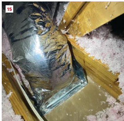
In the 2022 townhouse, the author's crew air sealed around the HVAC supply boots with canned foam (15, 16). In addition, the ducts themselves were sealed by the HVAC contractor using the Aeroseal system.
