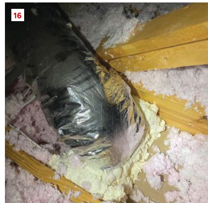
In the 2022 townhouse, the author's crew air sealed around the HVAC supply boots with canned foam (15, 16). In addition, the ducts themselves were sealed by the HVAC contractor using the Aeroseal system.
