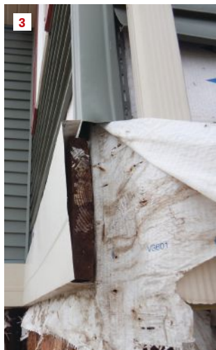
The capping of the band between siding types did not have an upturned leg (3). Without one, water drained into the wall. The lack of a kickout flashing (4) kept the corner of the garage framing soaked.
