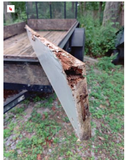
The existing frame-and-panel trim under the clad casement windows was fashioned from \frac{5}{4} pine and \frac{3}{8} -inch-thick plywood panels (1). Most of the rot occurred along the top edge of the horizontal trim members (2). The full extent of the damage could be seen after the author removed the trim (3, 4).
