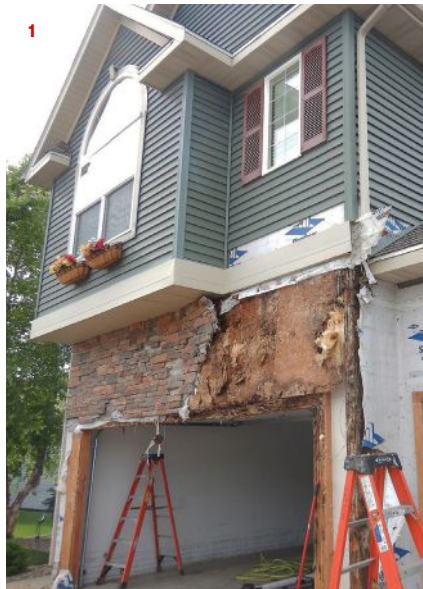
Mistakes with the WRB, the coil stock capping the band between siding types, and the flashing above the garage door led to the complete destruction of the sheathing above the garage door (1), turning the sheathing and LVL header into compost (2).
