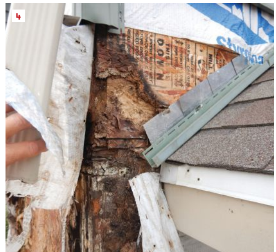
The capping of the band between siding types did not have an upturned leg (3). Without one, water drained into the wall. The lack of a kickout flashing (4) kept the corner of the garage framing soaked.
