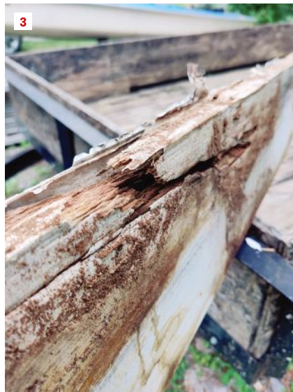
The existing frame-and-panel trim under the clad casement windows was fashioned from \frac{5}{4} pine and \frac{3}{8} -inch-thick plywood panels (1). Most of the rot occurred along the top edge of the horizontal trim members (2). The full extent of the damage could be seen after the author removed the trim (3, 4).
