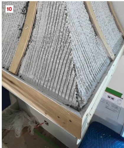
With the lower face complete and the boards to simulate the finish trim in place, a plasterer applies poly to protect the fan insert (6), then applies the metal lath (7, 8). Note the lath detail at the “hips” that prevents the cut edge of the lath from poking through the scratch coat (9). A plasterer then applies a scratch coat of plaster between the “ground” strips (10, 11).
