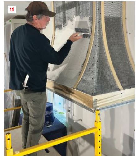
With the lower face complete and the boards to simulate the finish trim in place, a plasterer applies poly to protect the fan insert (6), then applies the metal lath (7, 8). Note the lath detail at the “hips” that prevents the cut edge of the lath from poking through the scratch coat (9). A plasterer then applies a scratch coat of plaster between the “ground” strips (10, 11).
