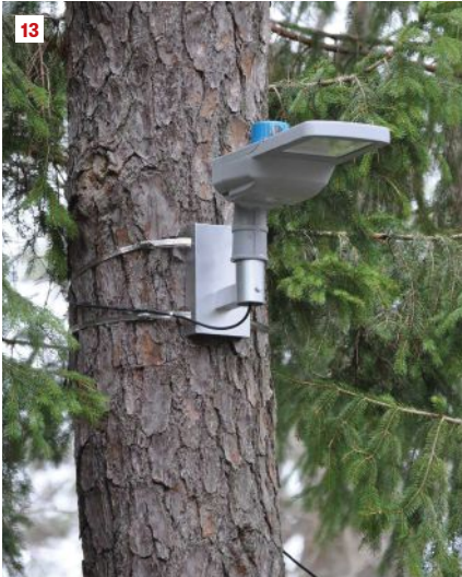
Light and motion sensor. The author mounted the brackets holding the LED light fixture (13) and motion sensor (14) on the tree with stainless-steel straps. The motion sensor is positioned lower on the trunk, which stands about 12 feet from the old utility pole on which the control box is mounted.
