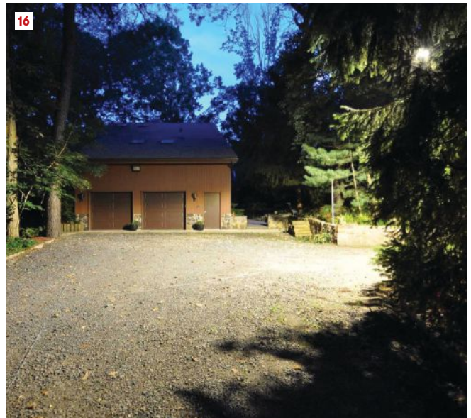
Results. Before the utility company took down the old mercury vapor lamp, the author had a chance to compare the light output of the old and new lights (at right and left in the photo, respectively) (15). The new LED successfully illuminated the area in front of the garage as well as the head of the driveway (16).
