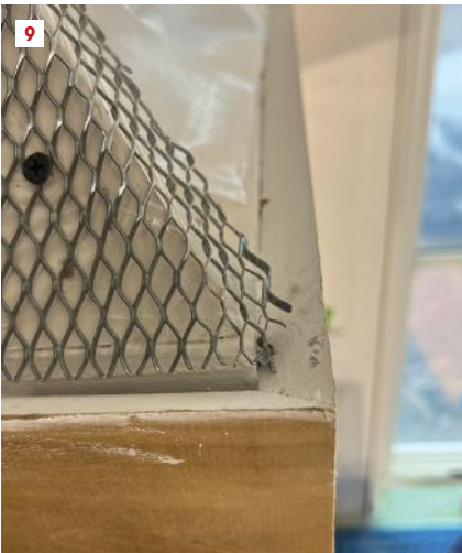
With the lower face complete and the boards to simulate the finish trim in place, a plasterer applies poly to protect the fan insert (6), then applies the metal lath (7, 8). Note the lath detail at the “hips” that prevents the cut edge of the lath from poking through the scratch coat (9). A plasterer then applies a scratch coat of plaster between the “ground” strips (10, 11).
