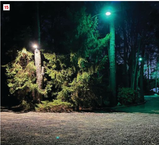
Results. Before the utility company took down the old mercury vapor lamp, the author had a chance to compare the light output of the old and new lights (at right and left in the photo, respectively) (15). The new LED successfully illuminated the area in front of the garage as well as the head of the driveway (16).
