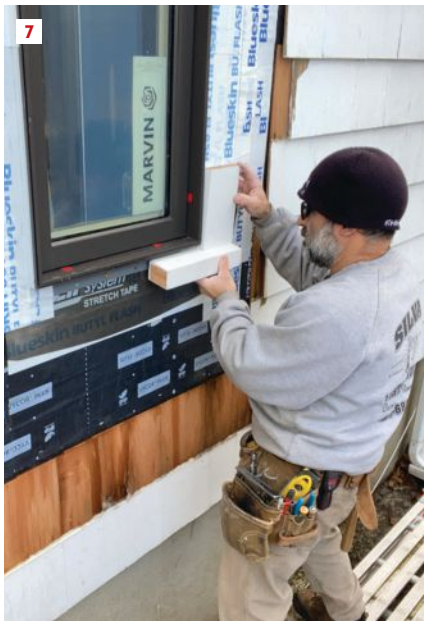
By making a mock-up of the sill and casing, the author is able to draw accurate lines to indicate where the components will be installed (7). Using those lines, he marks the header and sill for spacing and final lengths and then sizes the vertical parts that need to be cut (8, 9).
