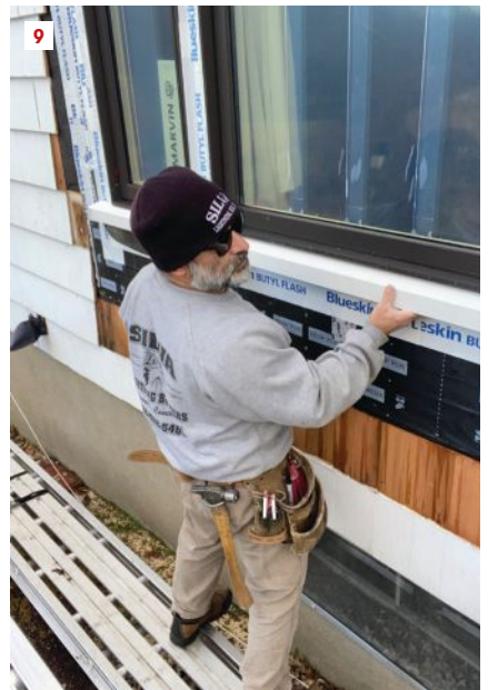
By making a mock-up of the sill and casing, the author is able to draw accurate lines to indicate where the components will be installed (7). Using those lines, he marks the header and sill for spacing and final lengths and then sizes the vertical parts that need to be cut (8, 9).
