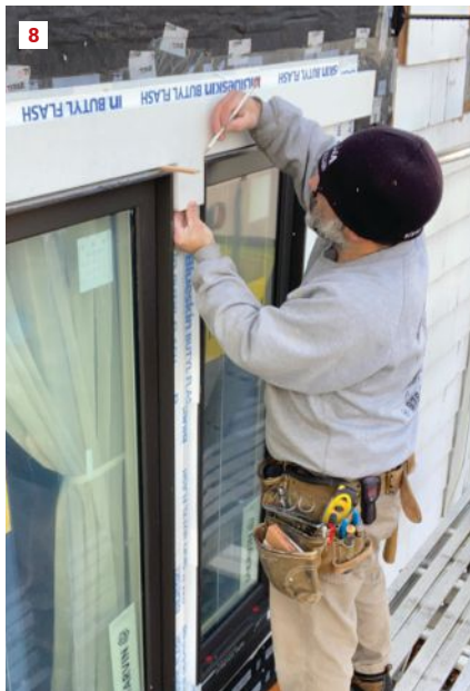
By making a mock-up of the sill and casing, the author is able to draw accurate lines to indicate where the components will be installed (7). Using those lines, he marks the header and sill for spacing and final lengths and then sizes the vertical parts that need to be cut (8, 9).
