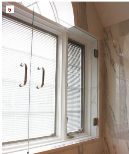
One of the last components to install is the first line of defense against splashing water: The author's company has the shower glass subcontractor fabricate hinged glass panels to cover the window (5, 6).
