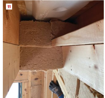
The resilience and consistency of TimberBatts allow you to sculpt them around the curves and angles of pipes (9, 10) with satisfying precision. The integrity of the fibers affords a high degree of precision fitting into odd-shaped framing cavities, such as this ceiling bay (11), but all this artistry comes at the cost of time.
