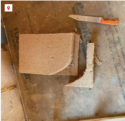
The resilience and consistency of TimberBatts allow you to sculpt them around the curves and angles of pipes (9, 10) with satisfying precision. The integrity of the fibers affords a high degree of precision fitting into odd-shaped framing cavities, such as this ceiling bay (11), but all this artistry comes at the cost of time.
