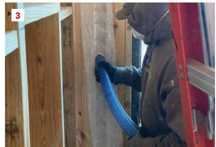
TimberFill. To avoid bulging bays when dense-packing walls, the author "lip-stitches" the membrane on the stud faces to pull it extra tight (1). On a different job, insulated mostly with batts, the crew needed to staple the membrane over odd cavities unsuited to batts (2) prior to dense packing them (3).
