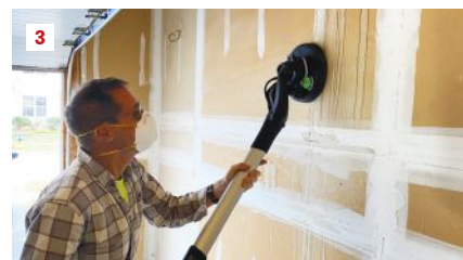
Garage walls yellowed from time and light and marred by water stains, dirt, and failing tape joints are a too common sight for the author (1, 2). To fix the surfaces, he starts by sanding them to clean and prepare the drywall for the next steps (3).
