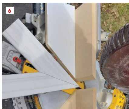
The illustration (top) shows a simple wall layout for applied molding. This same layout could be used with raised panels with added layers of trim elements. A site-built jig to cut angles above 45 degrees is affixed to the saw fence. Cutting a 45 on the end of the board first (5) makes getting sharper miters (6) easier.
