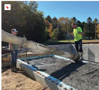
Shallow foundation. The new slab-on-grade additions were constructed with shallow frost-protected foundations.
