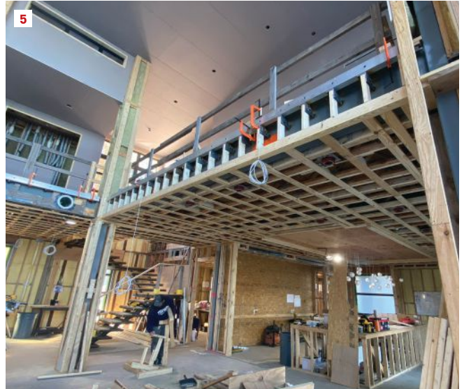
Once the rail supports are fixed to the I-beam (4), the crew frames out blocking and straps the ceiling below the balcony (5) and finishes the beam with plywood (6). To secure a glass panel in its aluminum channel, an installer uses a ratchet to tighten Taper-Loc shims, which had been inserted between the glass and the channel (7).
