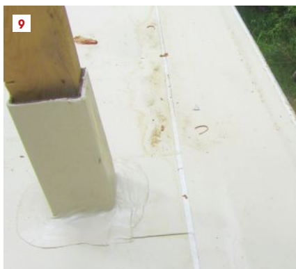
Preset sleeves. On this job, the guardrail posts drop into sleeves welded to the steel substructure (8). The sleeves are then waterproofed (9) and will be topped with a setting bed and limestone walk surface.
