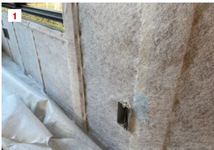
TimberFill. To avoid bulging bays when dense-packing walls, the author "lip-stitches" the membrane on the stud faces to pull it extra tight (1). On a different job, insulated mostly with batts, the crew needed to staple the membrane over odd cavities unsuited to batts (2) prior to dense packing them (3).
