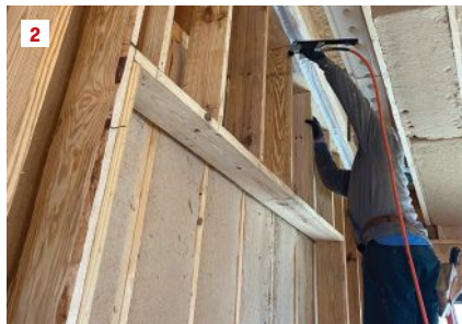
TimberFill. To avoid bulging bays when dense-packing walls, the author "lip-stitches" the membrane on the stud faces to pull it extra tight (1). On a different job, insulated mostly with batts, the crew needed to staple the membrane over odd cavities unsuited to batts (2) prior to dense packing them (3).
