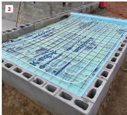
Shallow foundation. The new slab-on-grade additions were constructed with shallow frost-protected foundations.
