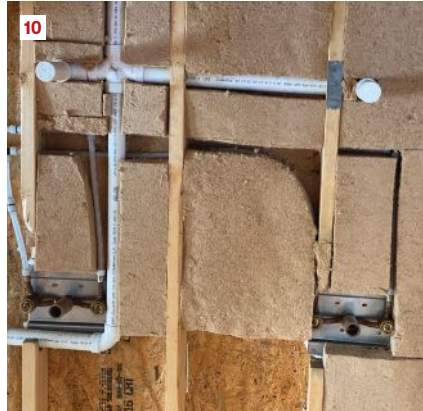
The resilience and consistency of TimberBatts allow you to sculpt them around the curves and angles of pipes (9, 10) with satisfying precision. The integrity of the fibers affords a high degree of precision fitting into odd-shaped framing cavities, such as this ceiling bay (11), but all this artistry comes at the cost of time.
