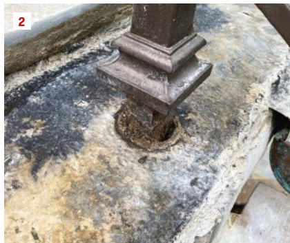
Efflorescence—white mineral deposits leaching out of stone and concrete (1)—is a clear sign of moisture moving through masonry, and its presence is helpful for identifying where a waterproofing layer has failed. The culprits here were the holes drilled through the waterproofing layer for the railing posts (2). To remedy this, the author's company removed the edge stone and waterproofed around the post bases (3).
