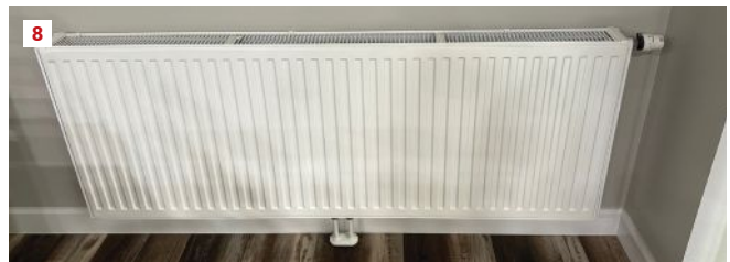
A SpacePak iLAHP cold climate air-to-water heat pump (6) is the home's primary heat source and also supplies chilled water for cooling. A 9-kilowatt electric boiler provides supplemental and backup heat (7). All Myson T6 panel radiators (8) have thermostatic control valves (in photo at upper right).
