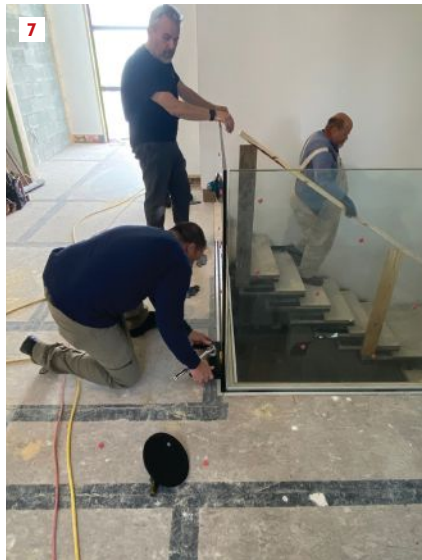
Once the rail supports are fixed to the I-beam (4), the crew frames out blocking and straps the ceiling below the balcony (5) and finishes the beam with plywood (6). To secure a glass panel in its aluminum channel, an installer uses a ratchet to tighten Taper-Loc shims, which had been inserted between the glass and the channel (7).
