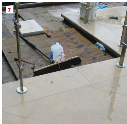
Preinstalled posts. The bases of these posts for glass railings needed to be bolted to the masonry deck (4, 5). The bases were waterproofed (6) and finished with stone and round escutcheon plates (7).
