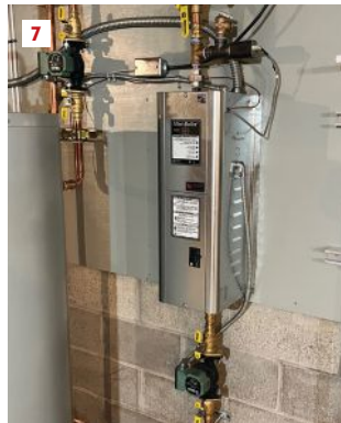
A SpacePak iLAHP cold climate air-to-water heat pump (6) is the home's primary heat source and also supplies chilled water for cooling. A 9-kilowatt electric boiler provides supplemental and backup heat (7). All Myson T6 panel radiators (8) have thermostatic control valves (in photo at upper right).
