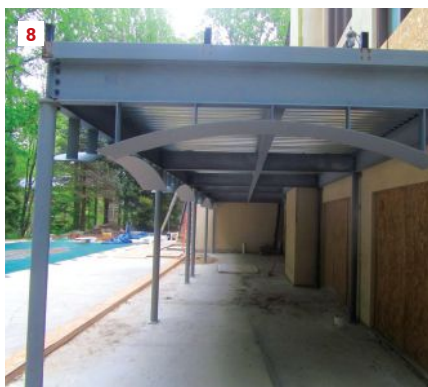
Preset sleeves. On this job, the guardrail posts drop into sleeves welded to the steel substructure (8). The sleeves are then waterproofed (9) and will be topped with a setting bed and limestone walk surface.
