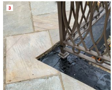
Efflorescence—white mineral deposits leaching out of stone and concrete (1)—is a clear sign of moisture moving through masonry, and its presence is helpful for identifying where a waterproofing layer has failed. The culprits here were the holes drilled through the waterproofing layer for the railing posts (2). To remedy this, the author's company removed the edge stone and waterproofed around the post bases (3).
