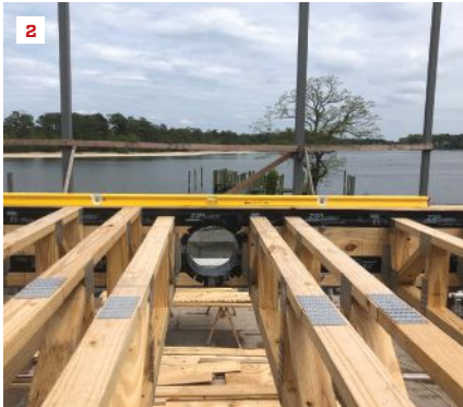
Running HVAC ducts in the open webs of floor trusses offers a distinct advantage. On this job, the truss layout (2) and the openings defined for ductwork in the trusses (3) had to be coordinated with prefabricated openings in the steel girders.
