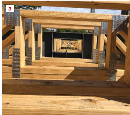
Running HVAC ducts in the open webs of floor trusses offers a distinct advantage. On this job, the truss layout (2) and the openings defined for ductwork in the trusses (3) had to be coordinated with prefabricated openings in the steel girders.
