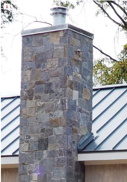
The photo above (1) shows a framed chimney clad with adhered stone. Details for the base flashing are shown in the illustration to the right of the photo. Details for the metal chimney cap are shown in the illustration on page 20.
