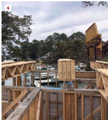
The author paints the top of wall plates blue to define duct pathways (4). At the edges of an area where trusses drop for a curbless shower, the author painted the top chord hot pink so framers stayed aware of a small change in elevation (5).
